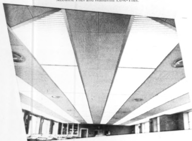
Suspended Ceiling to drawing office for The Workington Iron & Steel Co. Ltd., constructed from Corrugated Translucent Vinyl Sheetting with surrounds of Unitex Acoustic Tiles fixed by the MeTeO "C" Hook Metal Fixing System.
