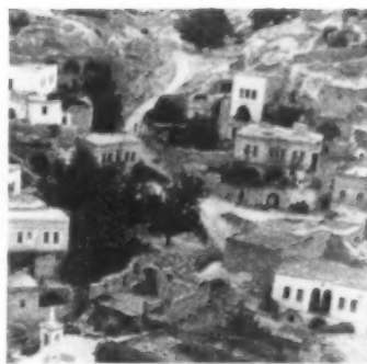
In the towns of the soft-rock area of Cappadocia, built architecture and excavated architecture are often inextricably mixed up in the same street, the same house. This view of a part of Keromeh, near Nevsehir, shows constructed fronts on houses whose back parts are caves, and arched undercrofts that seem to be constructed extensions of the caves behind.
