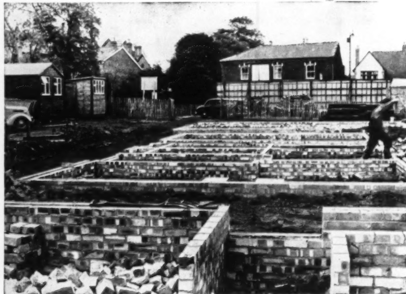
'Phorpres' Flettons being laid in foundations of the Birmingham Corporation Housing Development at Laurel Road, Handsworth, Birmingham
