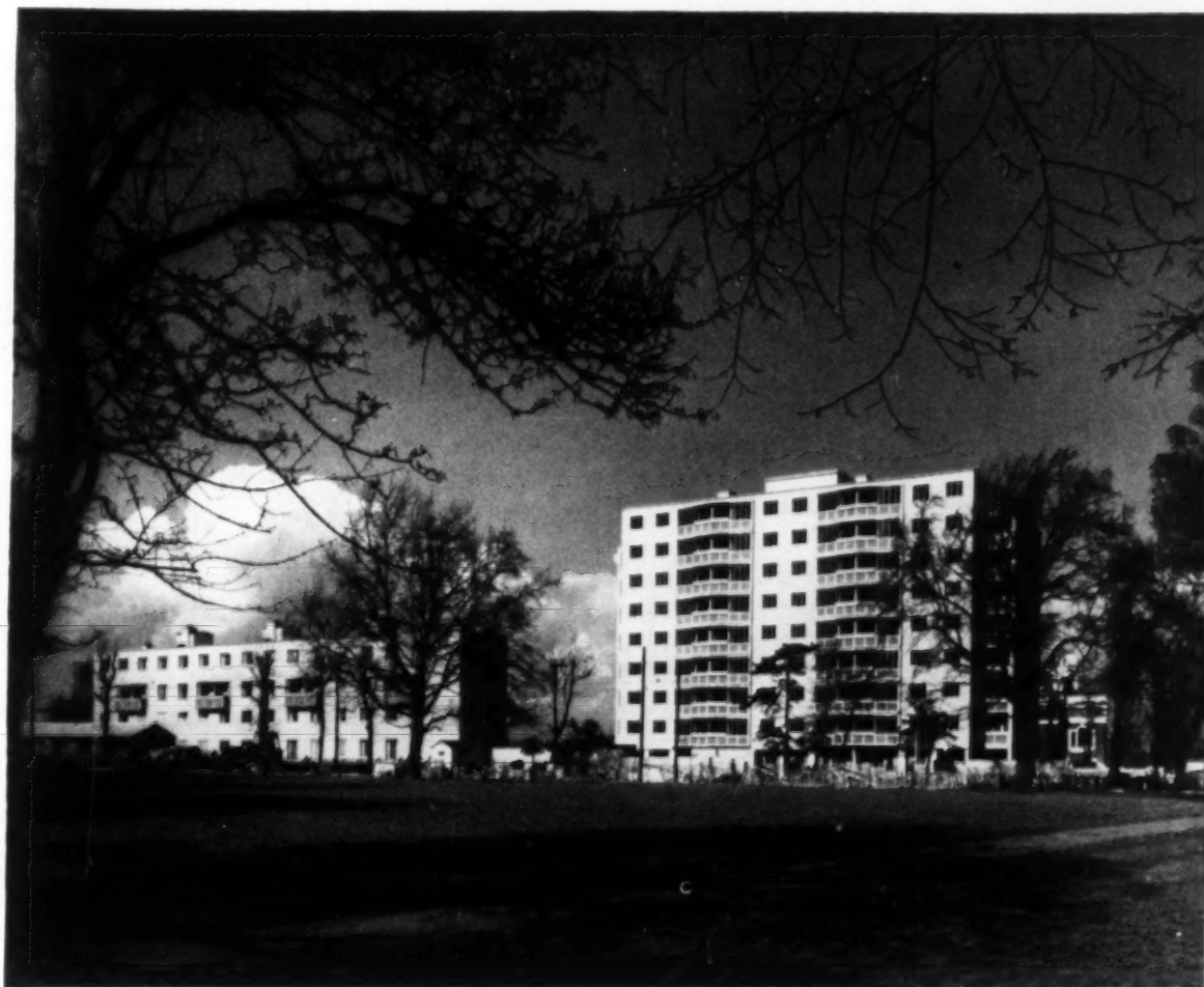
Tower Court Flats, Clapton Common
