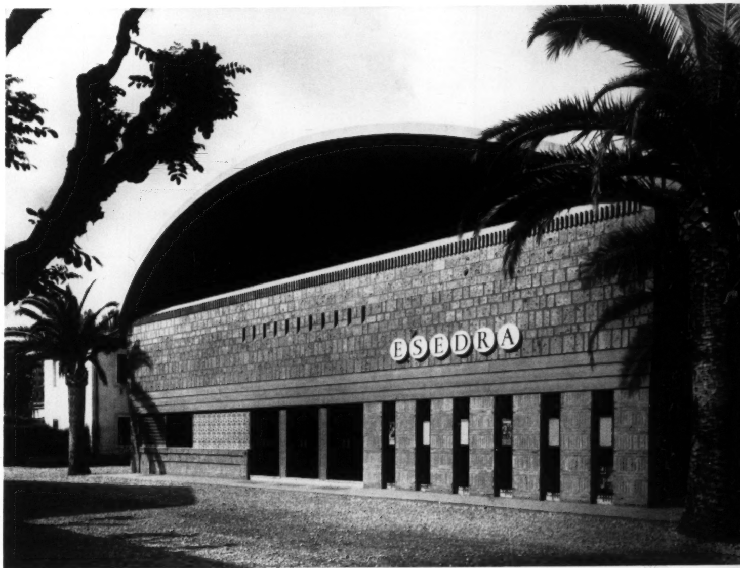
1 view of the facade.
