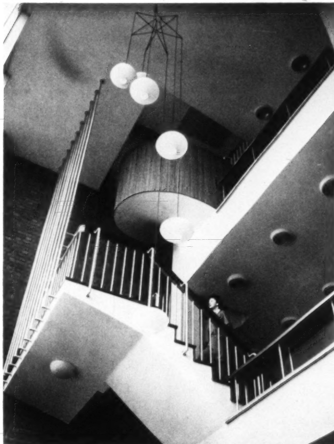
7, the main staircase, which forms the hub of the factory. The handrails are of aluminium, which is also used throughout the building for door furniture and partitions.
