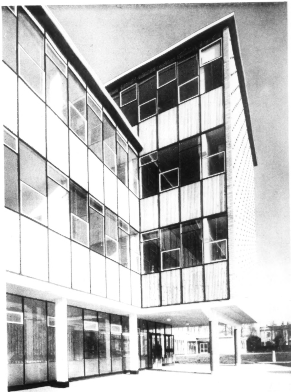
1. the main entrance; the panels below the windows are of red cedar, and the end wall is of rustic facing bricks. The two columns on the right are faced with narrow teak boarding.
