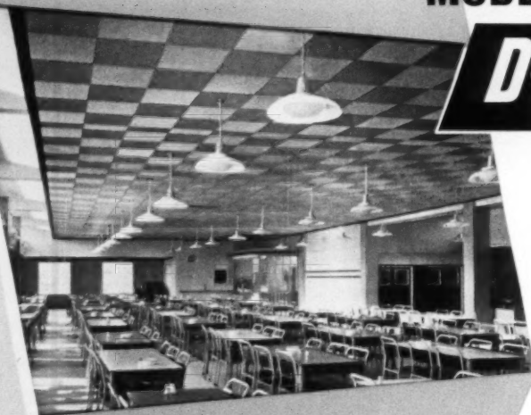
Burgess-Sulzer Heated Acoustical Ceiling, constructed from Burgess Acoustic Tiles in the Thortree Restaurant at the Wilton Works of Imperial Chemical Industries Limited.
