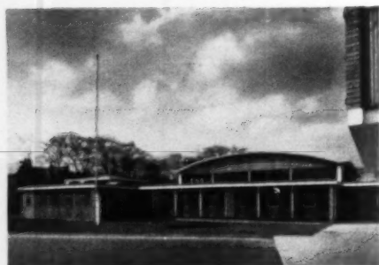
2, the assembly hall, from the main entrance.
