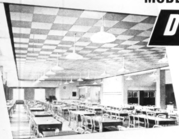
Burgess-Sulzer Heated Acoustical Ceiling, constructed from Burgess Acoustic Tiles in the Thorntree Restaurant at the Wilton Works of Imperial Chemical Industries Limited.
