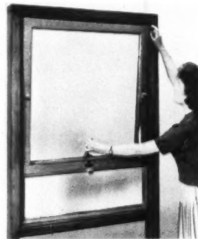
2. Releasing the casement
