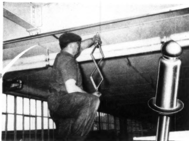
The photograph above shows 'Pop' Rivets being used for fixing suspended ceilings.
