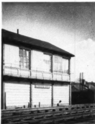
12, signal box at Mill Hill.
