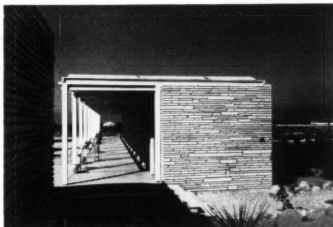
5. the marble slab wall at the end of the row of cubicles acts as a wind break.
