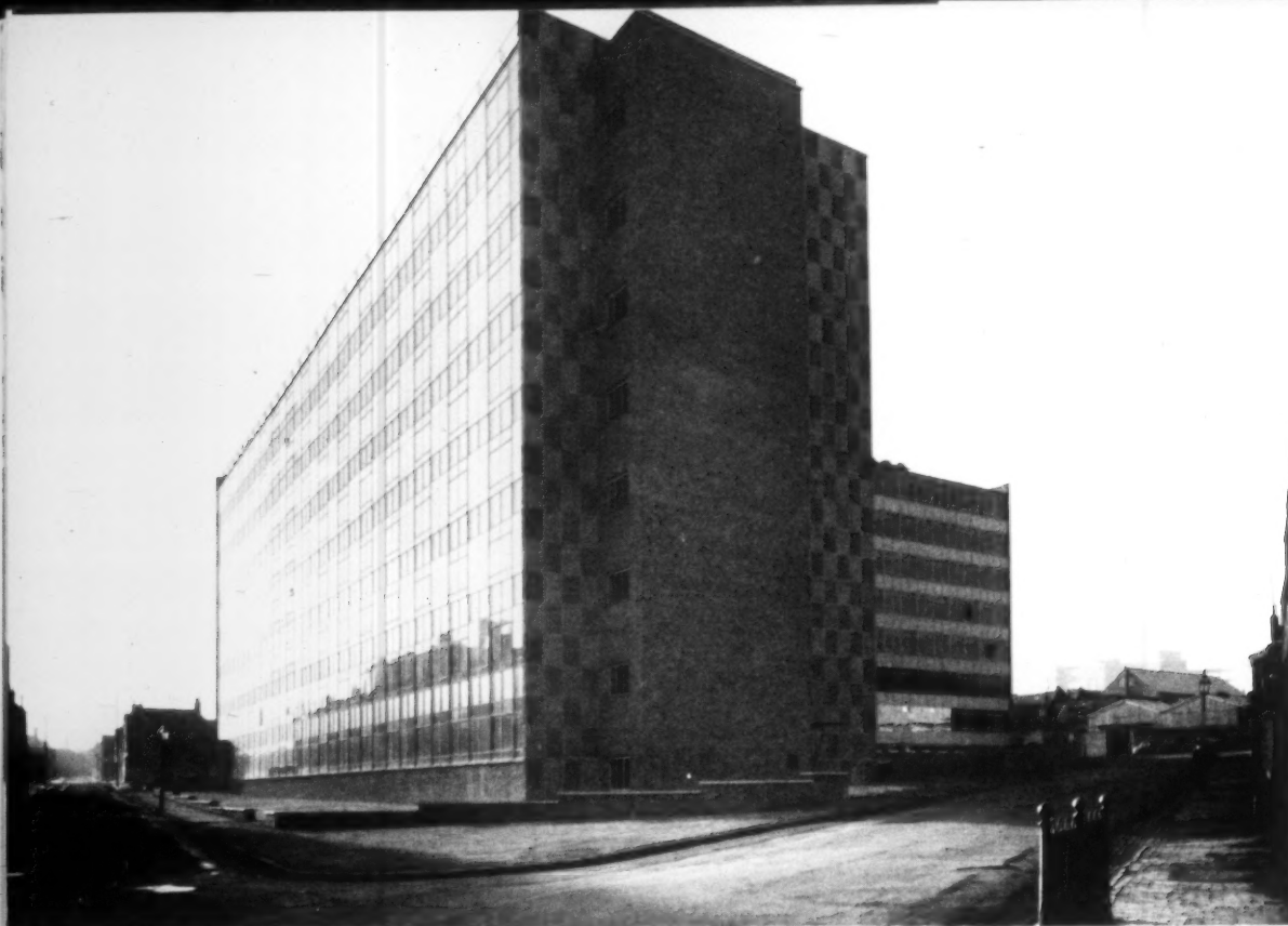
7, curtain walling on the north-east elevation.
