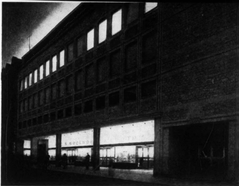
1, Sir William Holford's elevation to the new Woolworth's store, on the site of the old Clarendon Hotel, in the Cornmarket, Oxford.
