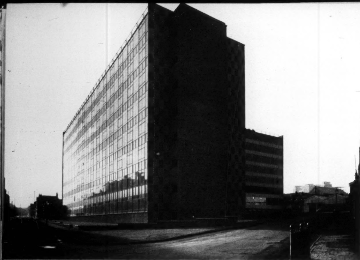
7, curtain walling on the north-east elevation.
