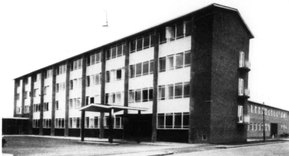
5, north façade and main entrance.
