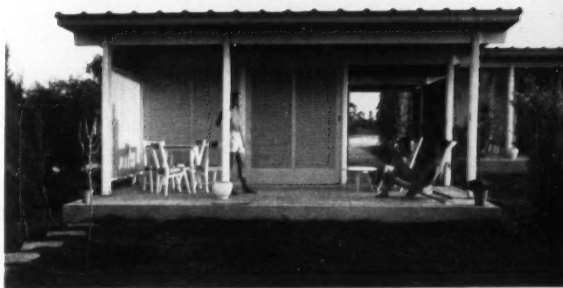
4 front view of a cabana, showing the louvred panels which can be folded back to open up the whole interior.
