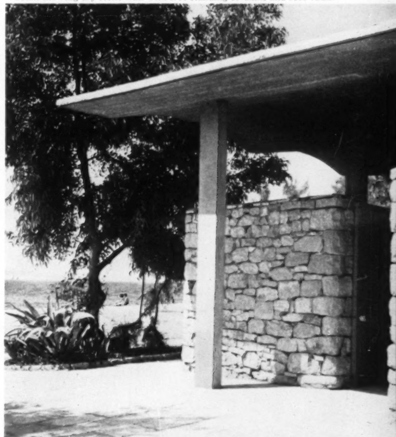
6. detail showing dry stone wall with free standing columns and roof vault.
