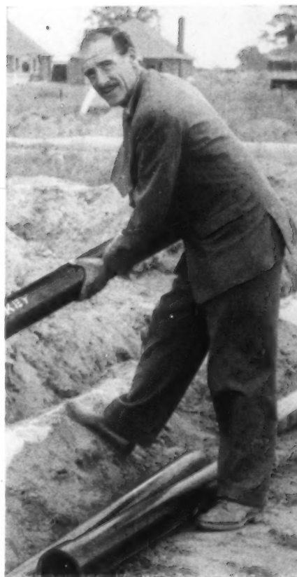
Major J. H. Hackett handling Key Pitch Fibre pipe on one of the building sites of his company.
