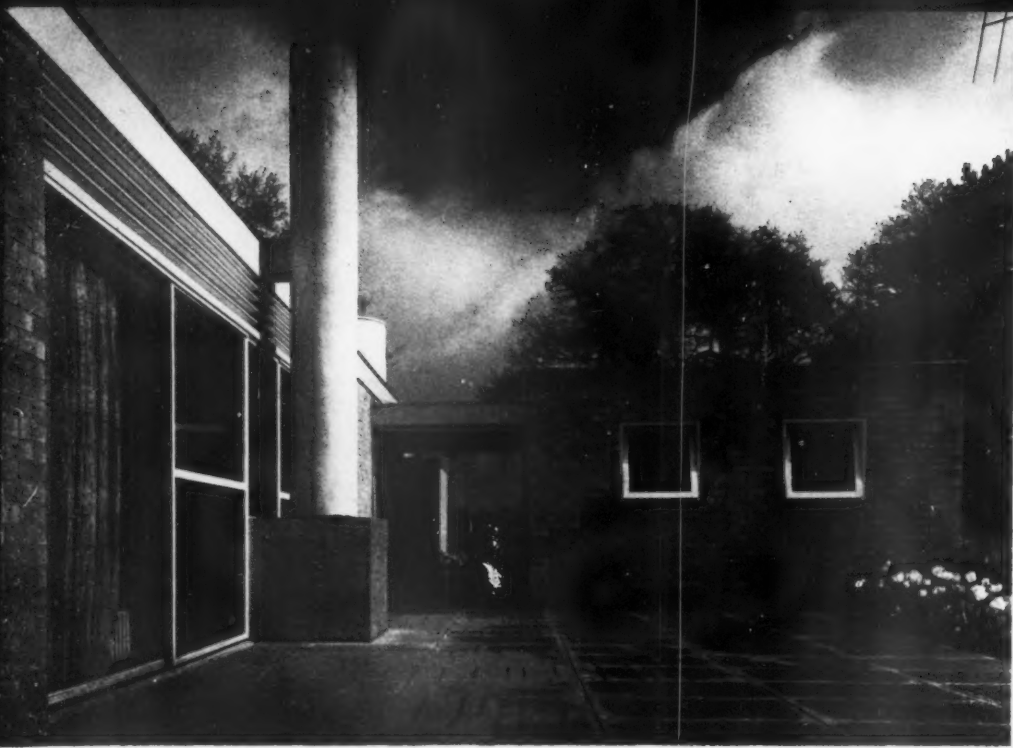
3, the north front, with the living room left and children's wing centre.
