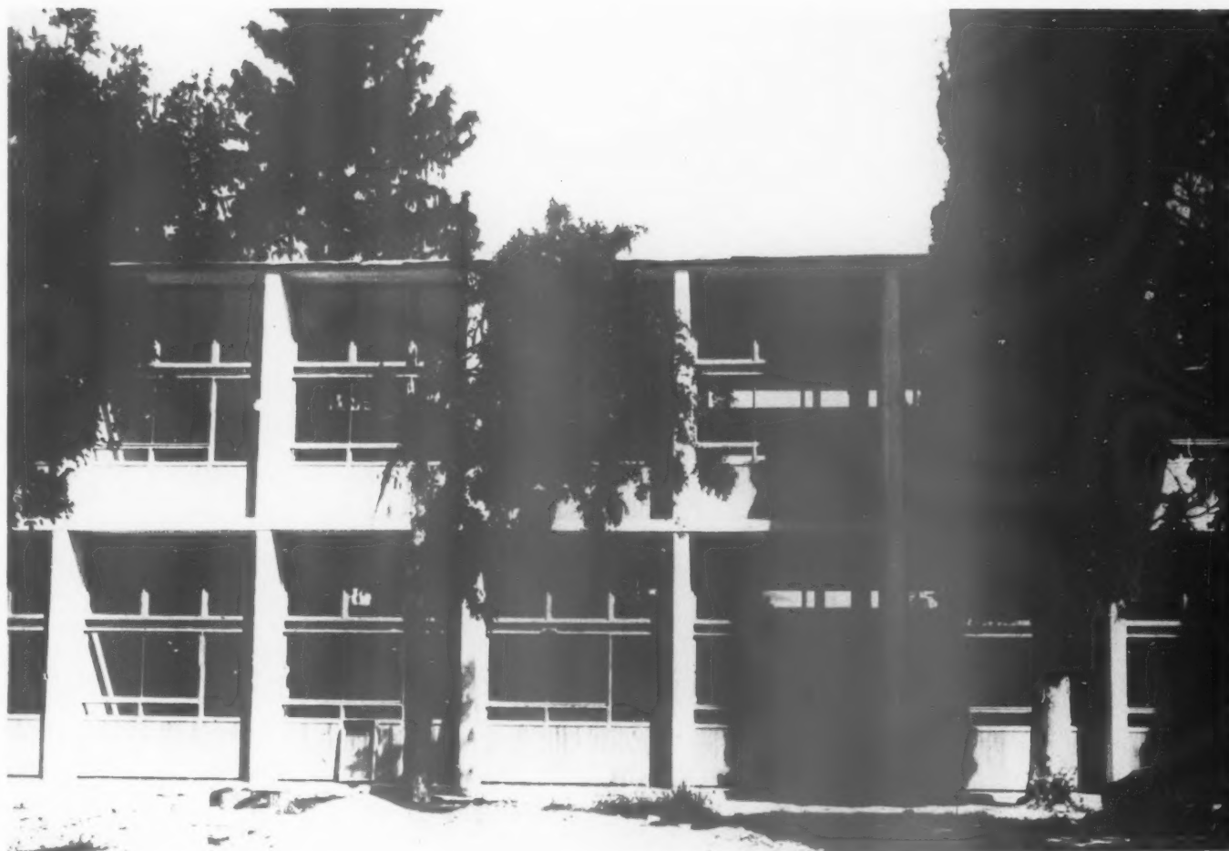
5, Ktima secondary school—progress view of classroom wing showing standard timber infill panels before insertion of horizontal shade hoods.
