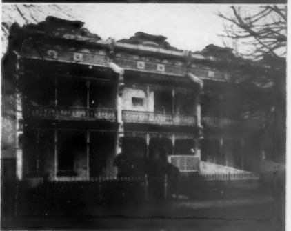
Four cast-iron Melbourne balconies; 1, offices in Victoria Parade; 2, St. Patrick's Boys' College; 3, house in Drummond Street, now painted mustard, black and white; and 4, a terrace at Carlton.
