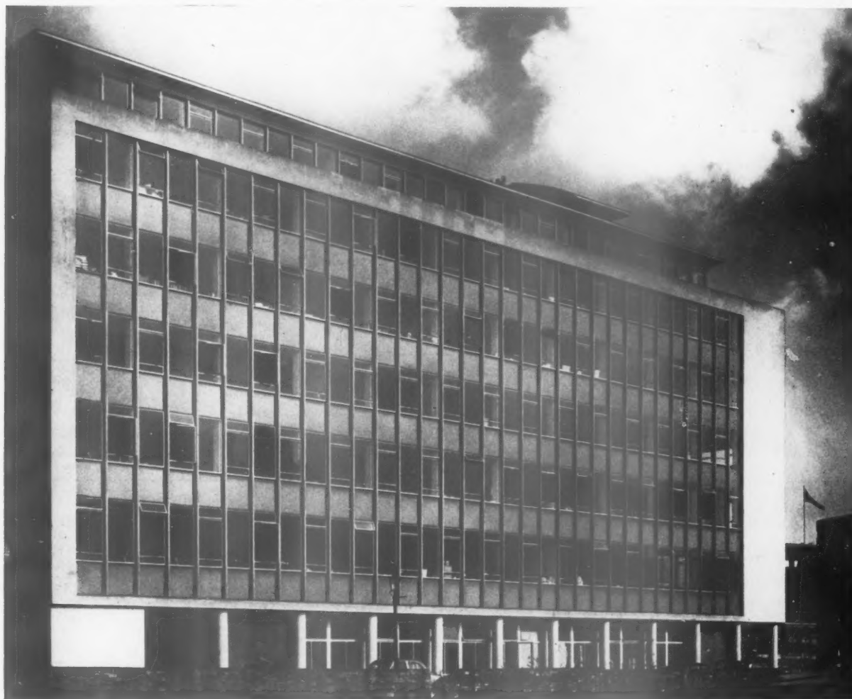
1, west elevation of offices, fronting Bunhill Row.
