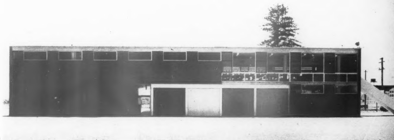
8. side elevation. The workshop area lies behind the steel doors on the right of the passage through.
