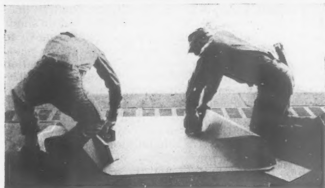
16, 17, typical of Fuller's adventures in materials, the Triennale dome of 1954, above, was built of units scored, folded and stapled up from sheets of standard packaging cardboard.
