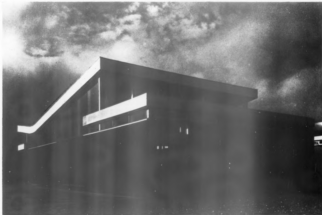
1, common room from the west. The roof is an 11½ in. timber roofing unit supported by a timber frame. The lower roof in the foreground covers the occupational therapy room and the store.
