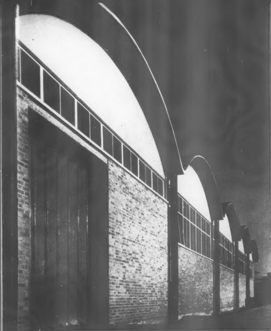
6, south front, with end of barrel roofing and folding metal doors, 7, entrance hall seen from opposite viewpoint to 5.
