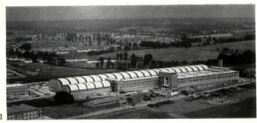
The printing works from the air. On the left, only half in the picture, is the canteen block. In the centre are the curved roofs of the large and small production halls, with the administration section alongside them.
