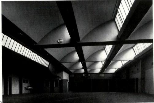
Above, some working-area interiors. 21, the main works entrance on the lower ground floor, with control turnstiles. 22, typical working space in the works section, with suspended ceilings and movable cross-partitions. 23, the general printing section showing the northlight roof, an independent construction cantilevered out from the columns framing a corridor on the right.
