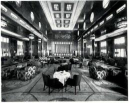
30, above, the Saxon, 1899, typical of the elaborate clerestories needed in earlier times for ventilation and light. 31, below it, the Queen Mary, with a clerestory 'hang-over,' now artificially lit, and not used for natural ventilation.
