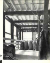
9, typical interior of intermediate floor in processing building; 10, the same in warehouse, each showing the fences of boards fixed to the flanges of the mullions, against which sacks can be stacked.
