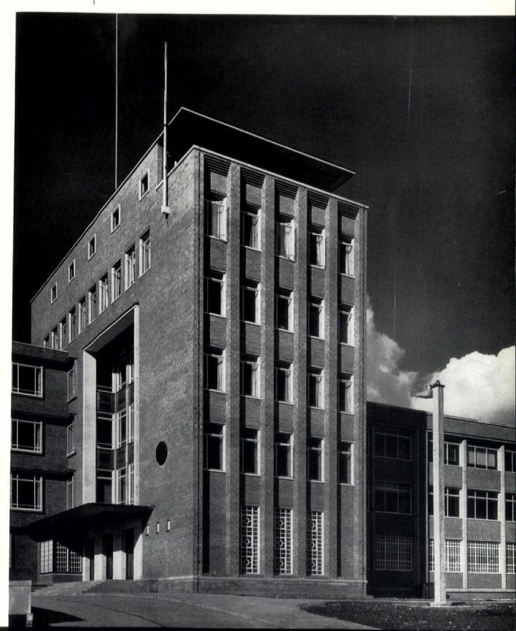
I, the main entrance of the administration section, which occupies the centre of the south front. The closely spaced glazing bars of the ground-floor windows were a security requirement. The brickwork is a brindled red. The reinforced concrete canopy has an undersurface of teak. The windows above are framed in Portland stone.
