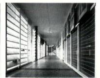
No. 31, which is a 3 in, by 1 in, mesh manufactured with 5 s.w.g. main wires and 10 s.w.g. cross wires. The panels are 6 ft. 8 in, high and 2 ft. 11 in, wide. The mesh was coated with anti-rust primer and painted three coats, and is secured with wood beads to a wood frame.
