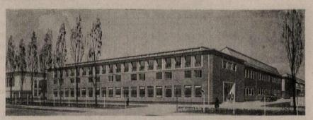
portion is formed by a series of aluminium portal frames, roofed with synthetic board covered with green mineral-surfaced felt. The production area only has a plenum ventilation and semi-airconditioning system, and the whole of the building is protected by a full sprinkler installation.
