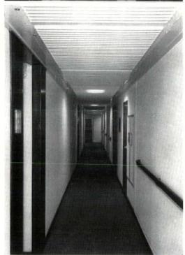
40, above, corridor in the Andes; apart from the reflecting walls which confuse rather than enlarge the space, and the unnecessarily elaborate trim to the door, it is further complicated by projecting ceiling lights, ventilators and fire sprays. 41, below it, on the Orsova, shows an ingenious way of overcoming this; an open false ceiling of statted-wood conceals all services and, since it is built in sections and hinged, provides easy access for repairs.
