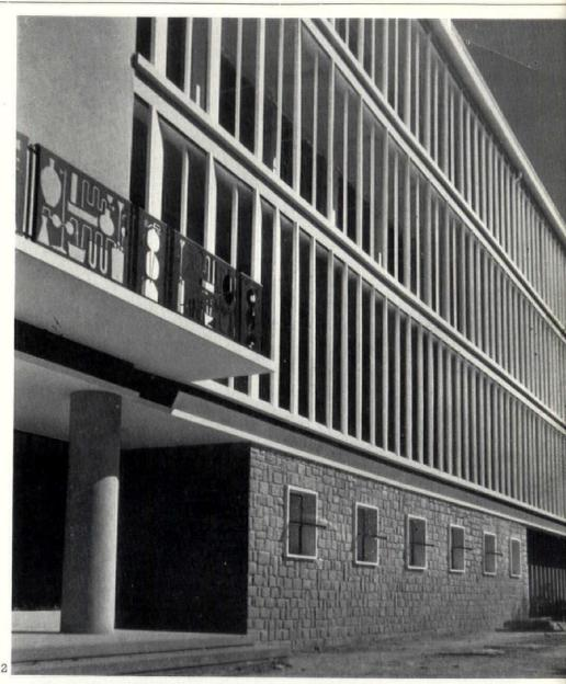
1. the entrance elevation. The vertical members are of concrete, with grey panels between of Shanghai plaster (see footnote on facing page). 2, the west side (see also distant views on facing page). The louvres, which act as sun-screens, are of concrete, plastered and coloured yellow with white edges. The ground - floor walls are of granite. 3, a detail of the design of the metal balustrade of the balcony over the entrance. It is painted dark blue.
