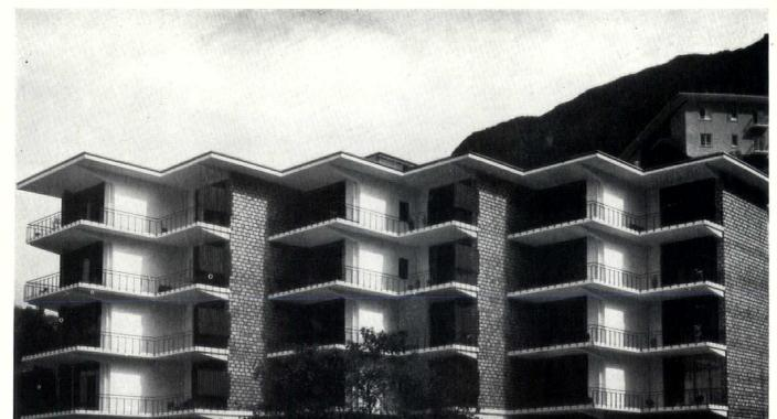
9, the west elevation. The main wall surfaces are granite and the others concrete, not plastered. It was a constricted site, owing to the precipitous nature of the university grounds, making an almost due west orientation unavoidable; hence the staggered plan, illustrated in this photograph.
