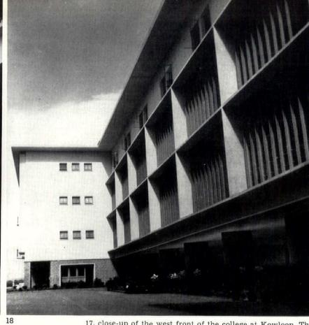
17, close-up of the west front of the college at Kowloon. The balcony is reached from the windows of the cafeteria The large window above lights a lecture hall. Materials are plastered concrete and local granite. 18, the entrance façade. Concrete louvres are green and the framing members white. The columns beneath are dark blue.
