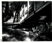
comes from Australia. The functional excuse here was a difficult site bisected by a creek which had to be left unencumbered; the structural solution evolved by its architects (Grounds, Romberg and Boyd) was an unusual one—to sling a singlestorey house of Miesian aspect and wedge-shaped plan between two lattice arches, grounded on massive
