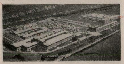
framing, which in the main is clad with aluminium sheet lined with insulation board. A plinth round the building is of precast concrete slabs. The south wall had to be constructed of brickwork with large metal windows, since it was required to match an adjoining building. The factory roof is an aluminium deck.
