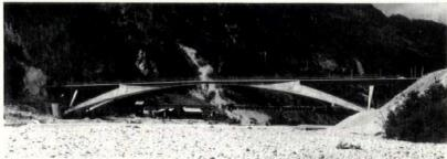
QUADRICABLE BRIDGE. Part of a remarkable project for feeding surplus furnace gases from the Saar into the urban supply net-work surplus furnace of Paris, over 300 km. distant, this bridge which carries the pipe-main
