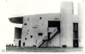
15, the normal entrance between two of the side chapels. Note the expansion joint between the chapel tower and the main wall.
