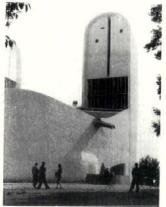
14, the side chapel towers are provided with a concrete grille which catches the sunlight at different times of day.
