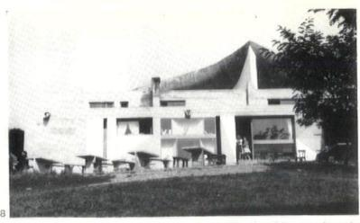
8, the chapel roof is seen above the hostel which is built throughout of in-situ concrete walls, incorporating timber and glass shelving units. Tables in the foreground are in precast concrete.
