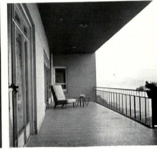
This building only was carried out in association with a Hong Kong architectural firm, Messrs. Chow and Lee. It occupies a steeply sloping site on the higher part of the University grounds, with views looking northwards over the harbour. It is a reinforced concrete frame structure, finished externally in the local granite (which is of good quality and light grey in colour) and plaster. The wood used externally (for balconies) and internally is teak.
