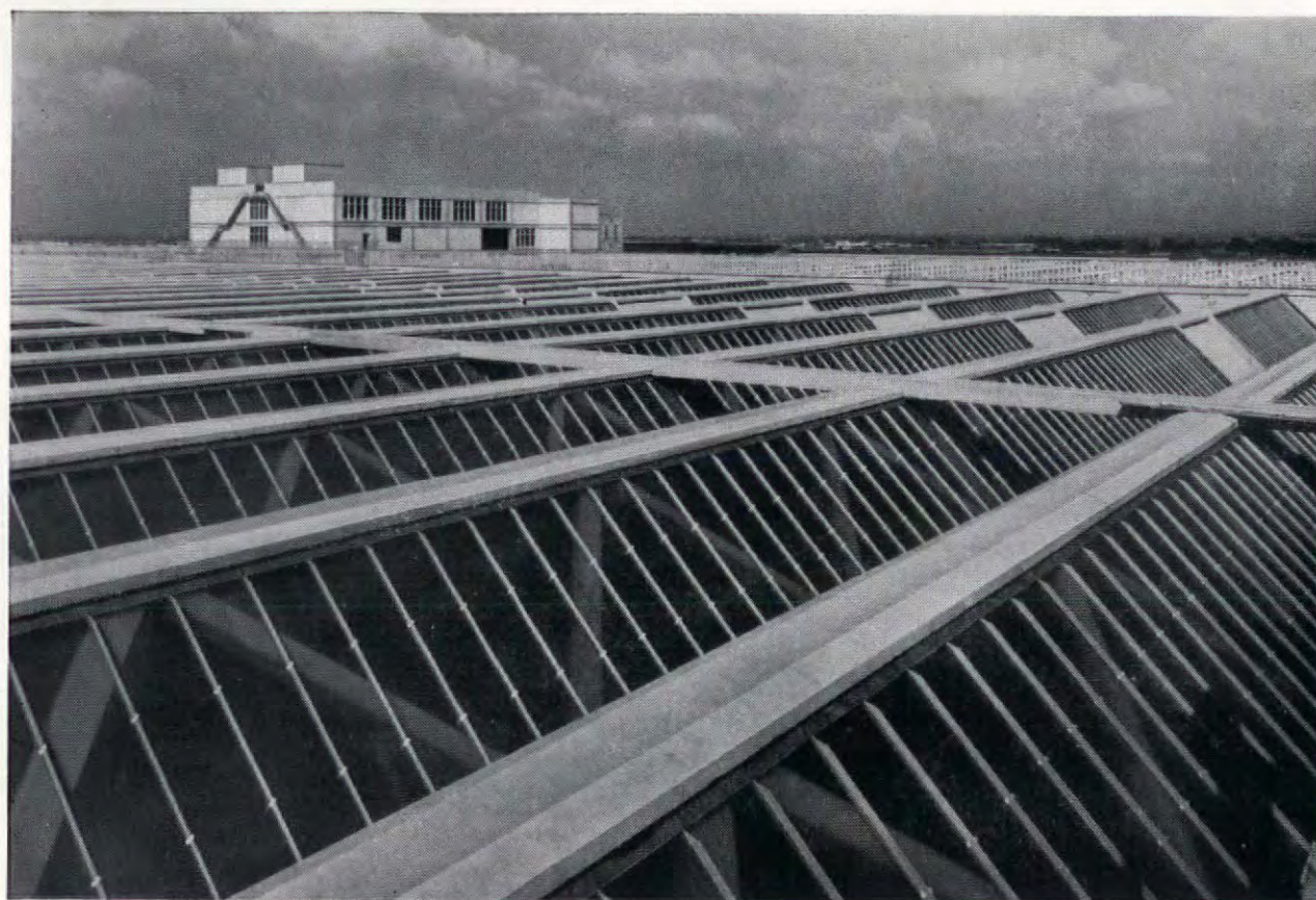
Part of the roof of the B.O.A.C. Headquarters at London Airport. The total area of glazing is approximately 280,000 square feet.
