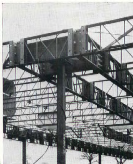
8, Boreham Wood Primary School (Herts CC). Detail of the Frameweld construction showing the adaptation of the column head to take the beams on the half module.
