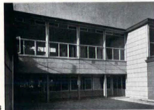
6, Bessemer Grange School, Denmark Hill (LCC): an example of the standard 8 foot 3 inches frame adapted for use in double storey construction.
