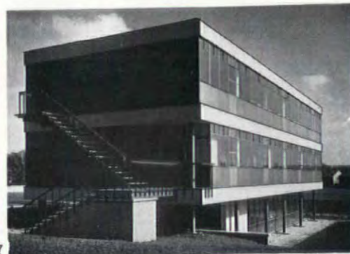
7, Oxhey Clarendon School (Herts CC) using Holoplast cladding on a Hills frame.
