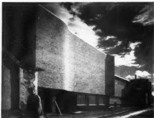
25, view along the west flank of the building, 26 and 27, the loading bay with cantilevered reinforced concrete canopy. The end wall seen on the right in 26 has a temporary finish, to allow for a future extension. 28, 29 and 30, on the facing page, views of the ventilator house on the east side of the building.
