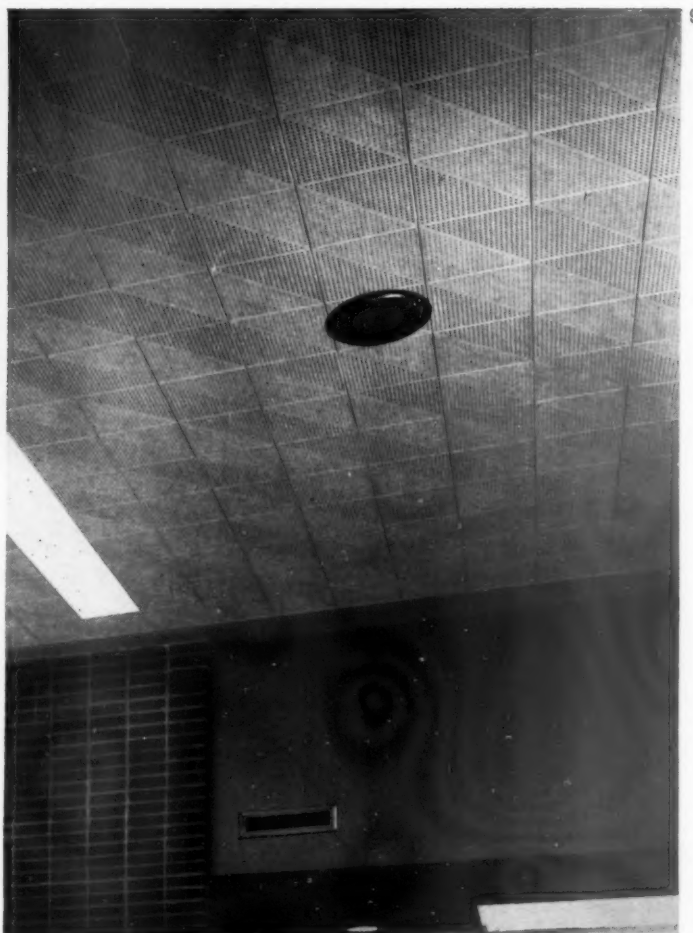
fibreboard 7, Tentest Rabbit Warren acoustic board. 8, Uniton tiles with irregularly spaced perforations. 9, Uniton mosaic tiles showing perforations of two different diameters.
