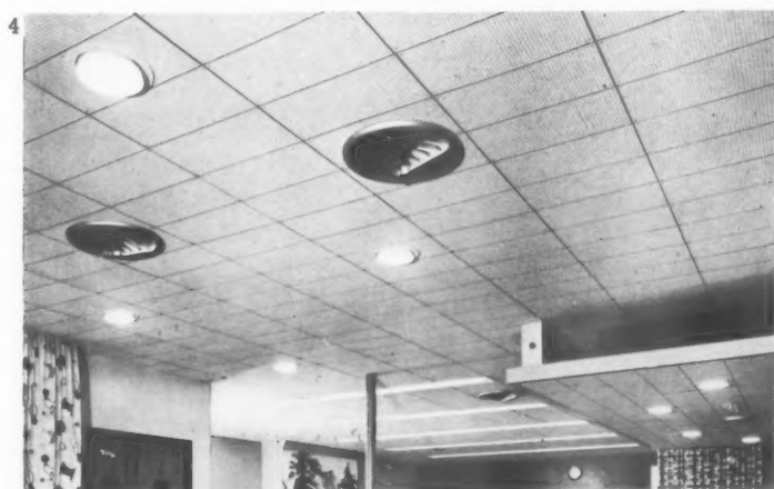
fibreboard 3 , the Cullum channel fixing system for forming suspended ceilings with acousti-celotex tiles. 4 , acousti-celotex perforated fibreboard tiles. 5 and 6 , Unitone tiles and their method of fixing.
