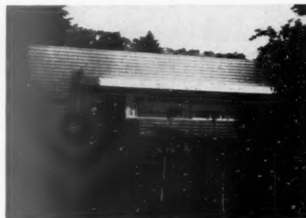
'Fural' aluminium sheeting on a house at Genfersee, Switzerland. (Architect: Le Corbusier).
