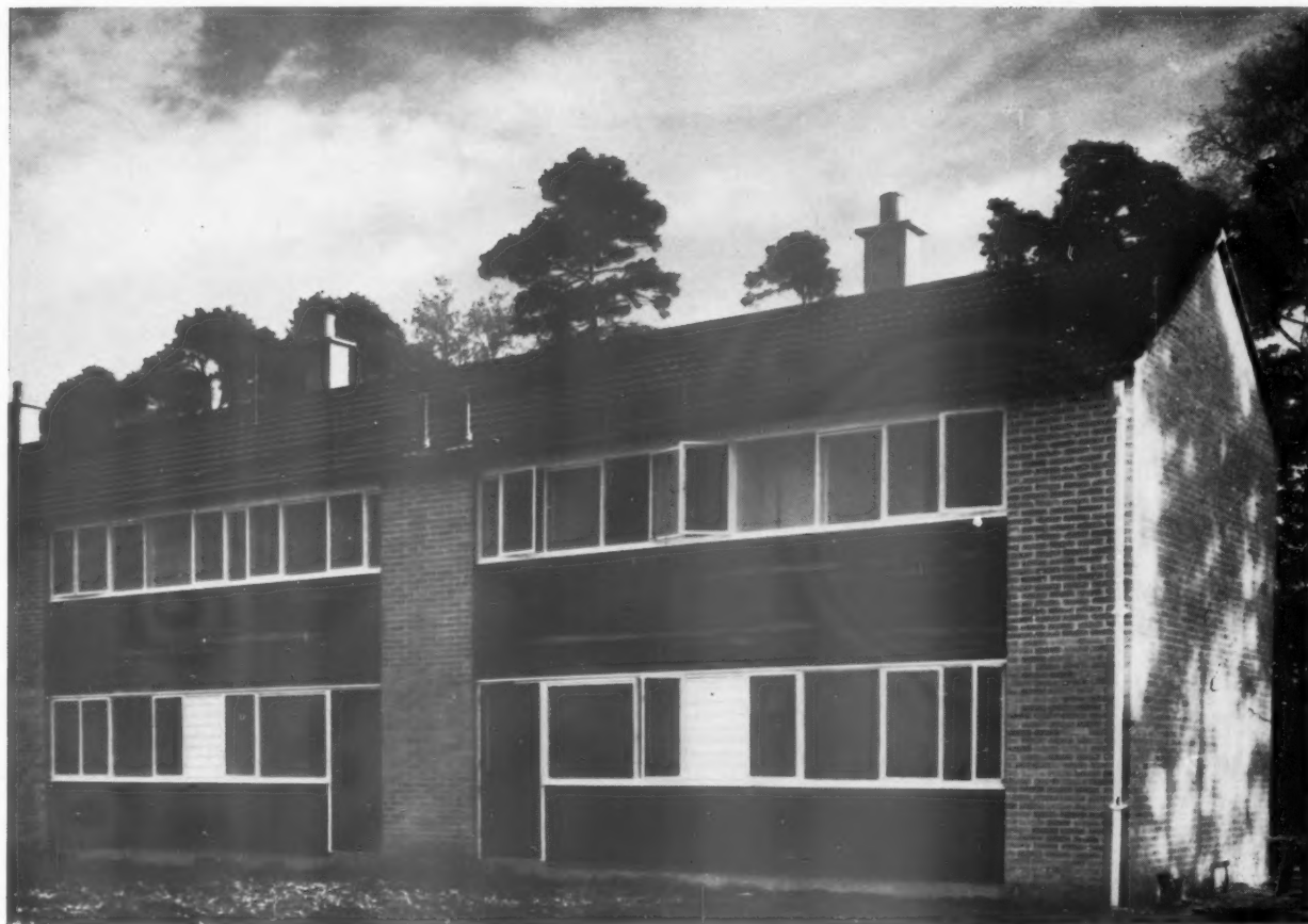
1, rear elevation part of the terrace of eight houses.
