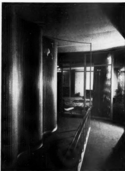
'Rollywood' on a curved internal wall at Sanderson's Three Arts Exhibition.
