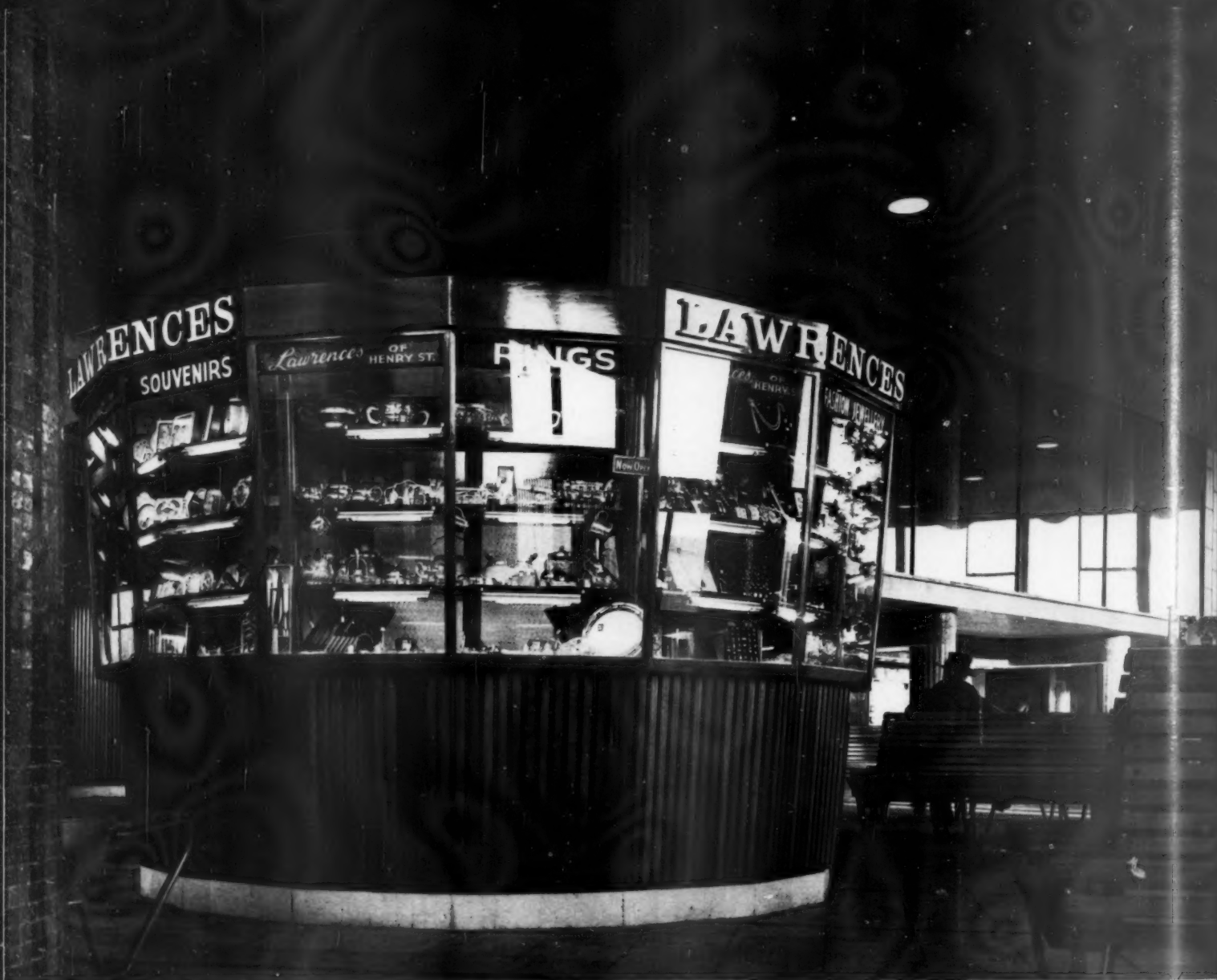
23, a kiosk in the central concourse. Timber slatting is mahogany. Columns in the concourse are finished with dark purple and grey mosaic.
