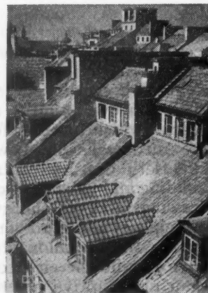
1, roofs of the rebuilt houses enclosing Warsaw's Old Town Square, showing artists' penthouse studios.
