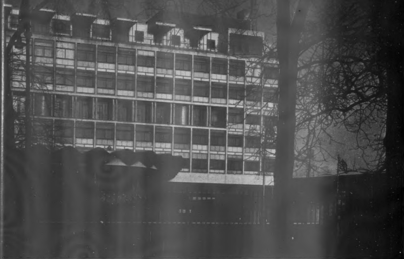
5, view of the office blocks at night. 6, the same view by day. Reinforced concrete structural members and end walls are faced with Portland stone: windows are set in bronze frames. 7, the six-storey block looking north. The decorative balcony expresses on the elevation the planning of the third floor as a suite for the Minister for Social Welfare. The setback of the penthouse restaurant provides an outdoor dining terrace.
