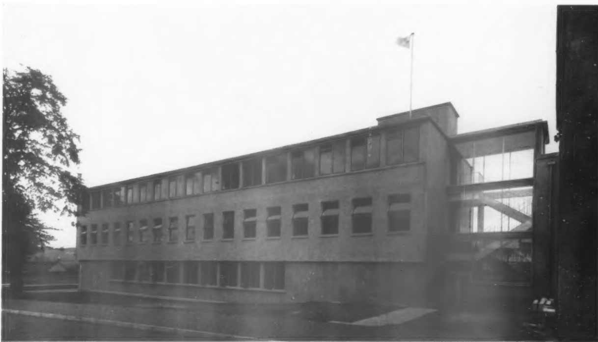
1, the new block from the north-east, showing covered staircase linking the old block to the new.
