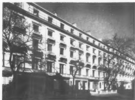
Cement paint on a terrace of flats in Bayswater. (The Adamite Co.)
