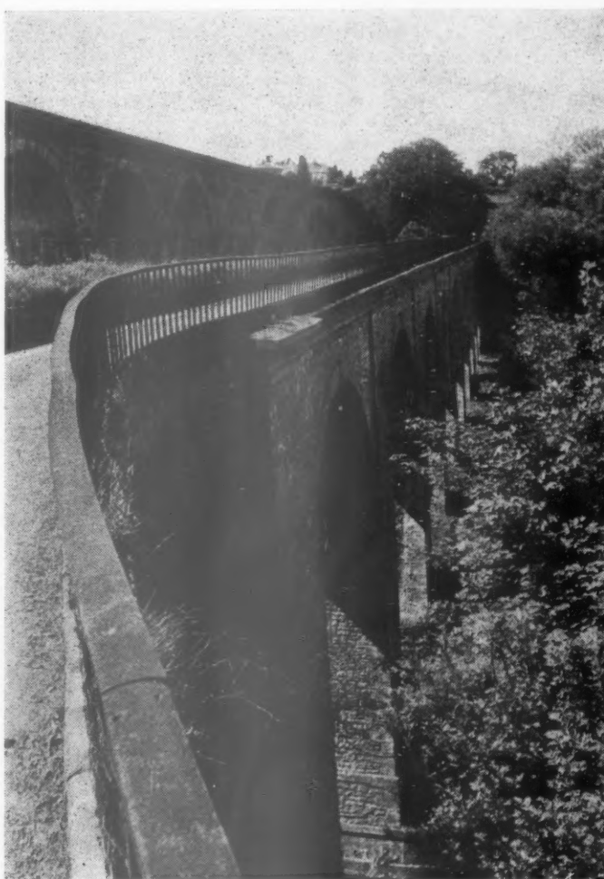
CHIRK This aqueduct has masonry piers and trough walls. Only the trough bottom is cast-iron. It lacks the grace of Pont Cysyllte, particularly in contrast with the grander railway viaduct, of a later date, standing beside it.
