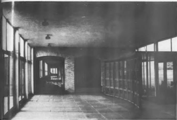
13, the main entrance hall looking north east. The passage on the left leads past cloakrooms to biology, music, woodwork and metalwork rooms.
