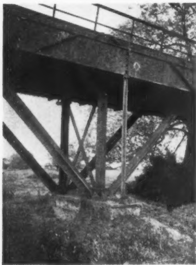
Telford's cast-iron aqueduct of 1795, the first of its kind, carrying the Shrewsbury canal over the River Tern.
