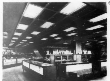
The flexible lighting system for John Walsh's rebuilt store.
