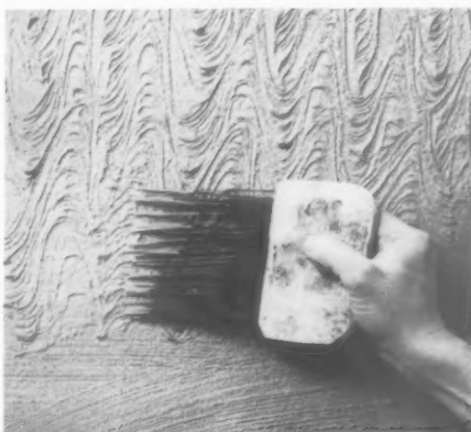
The texture produced by a line of stiff bristles embedded in a handle: similar effects can be produced with other tools such as brushes, corrugated rubber, or even with a loosely screwed up ball of newspaper. (The Cement Marketing Co.)
