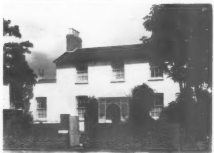
Exterior damp-proofing combined with decoration. One coat of primer and one finishing coat applied early in 1947. The house (at Strand-on-the-Green) photographed in August, 1953. (R.I.W. Protective Products Co.)
