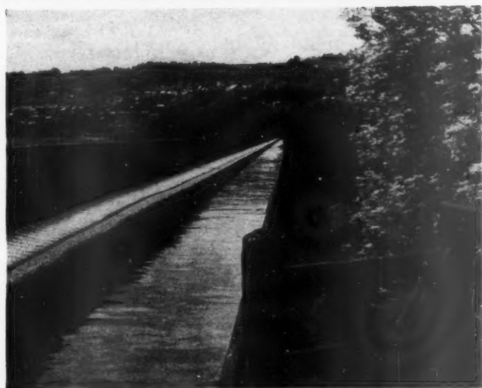
PONT CYSYLLTE 2, general view showing the extreme economy of materials used. The trough section has been reduced to a minimum: the masonry piers are hollow above the first 70 feet. 3, view at canal level. The towing path is placed over the water to reduce resistance to boats.
