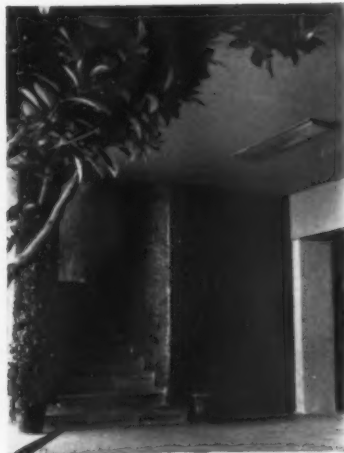
2, a staircase in the science block with mosaic facing.
