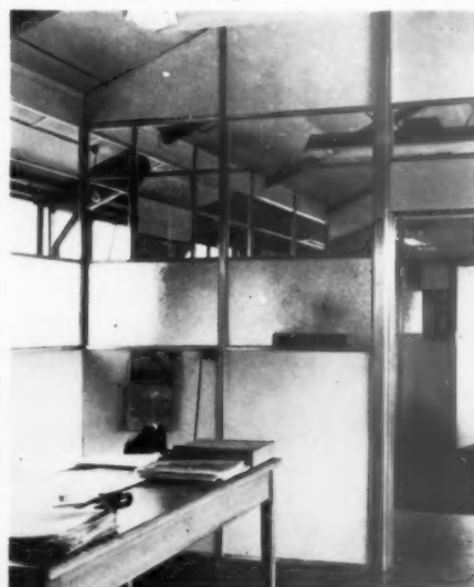
Offices in a temporary building at London Airport. The framework is in extruded aluminium sections and the panels are high density resin bonded chipboard. (British Plimber.)
