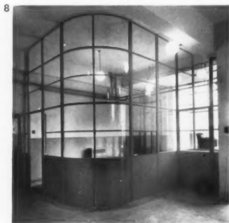
Office partition produced by a firm of window manufacturers. Standard glazing bars are used with tubular mullions to join the panels. The sheeting can be single, or doubled, and the space filled with insulating material. (John Williams.)
