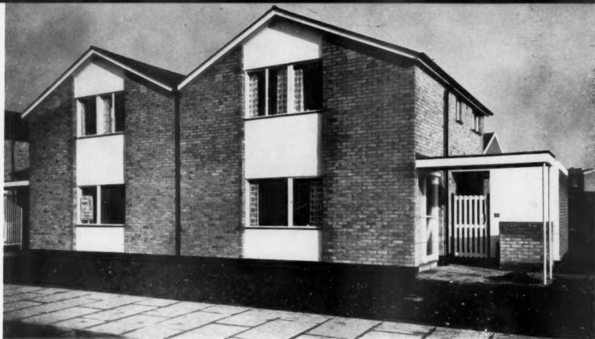
8, one pair of houses from the south-west.
