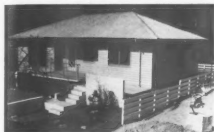
9, rear elevation of the Precut timber house.
