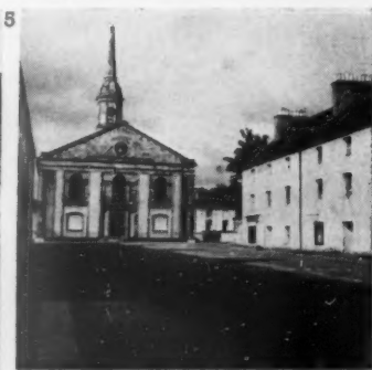
5, Main Street showing Mylne's three-storey tenements.
