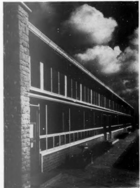
2, classroom wing from the west.
