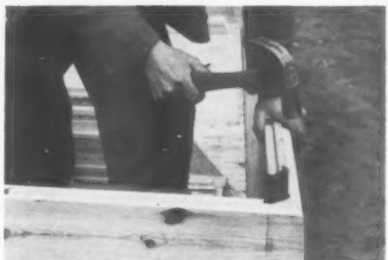
10, fixing the FRYA corner construction which binds the house together.
