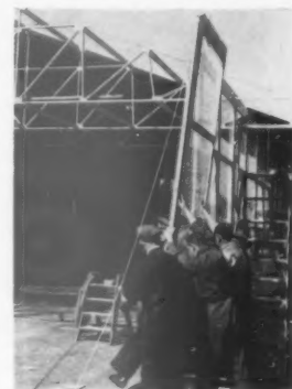
14, erection of wall panels of a Hawksley G.P. building.
