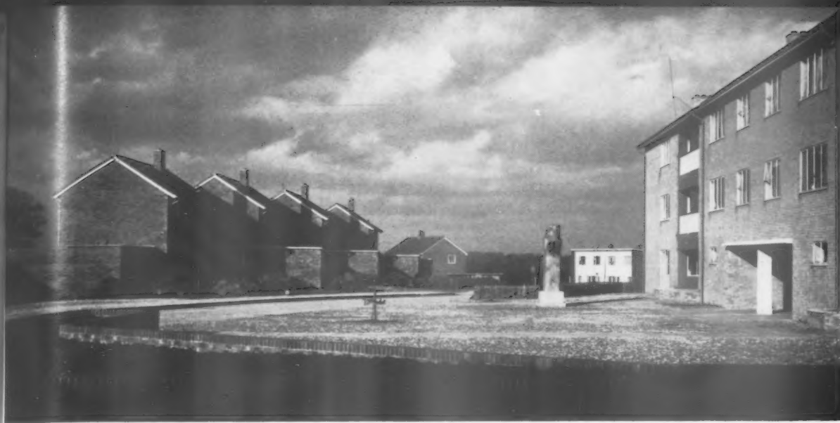
Detached houses on the left, seen from the south.
