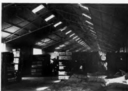
3, interior of Arcon storage building.
