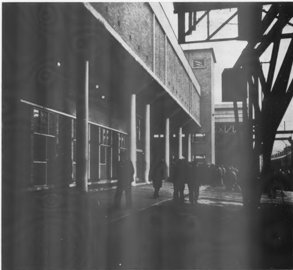
9. southern extremity of the drawing office block with the workers leaving the workshop area which runs down to the water front and moving up the concourse to the main shipyard entrance.
