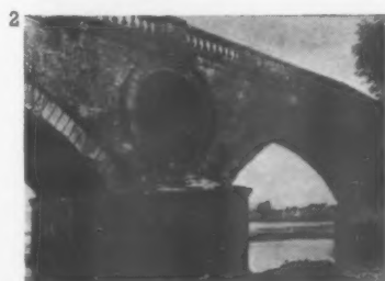
The Aray Bridge.
