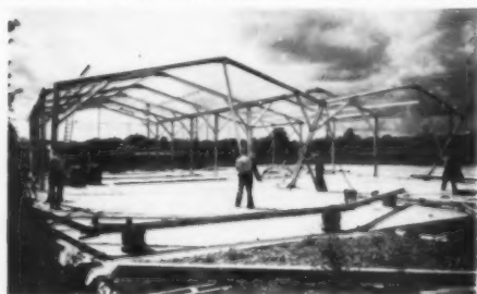
17, Alframe structural members being erected for garage building.
