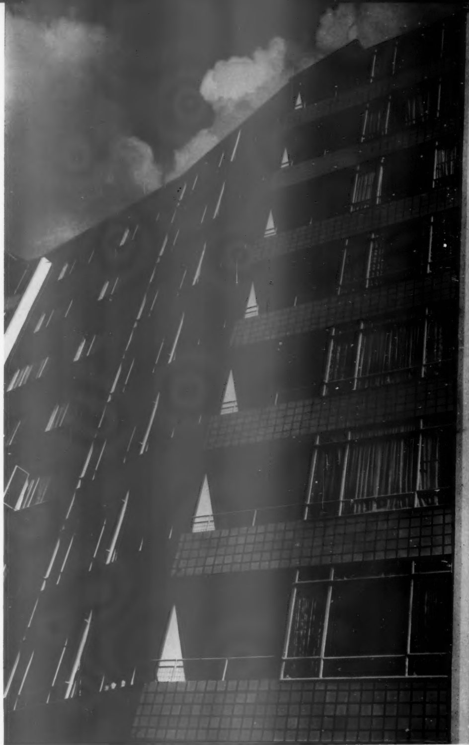
1, detail of the balconies of the eight-storey blocks. Balconies are faced with blue-grey tiles and recesses are blue, yellow or red. 2, view of the eight-storey blocks looking east from the terrace over the shops that face King's Road.
