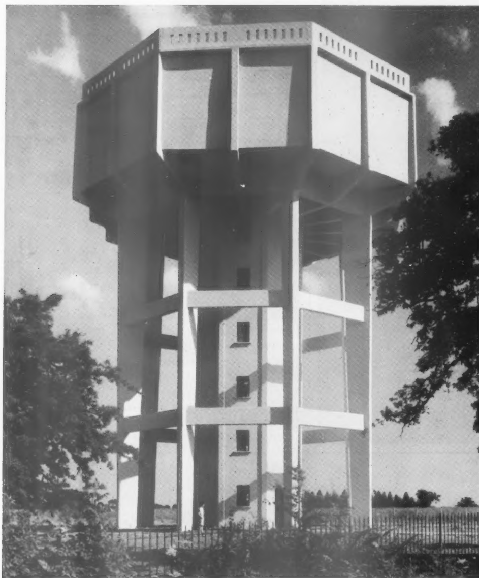
Reinforced Concrete Water Tower at Stowlingtoft for Thingoe and Thedwastre R.D.C., Consulting Engineers: Messrs. Lemon & Blizard.
