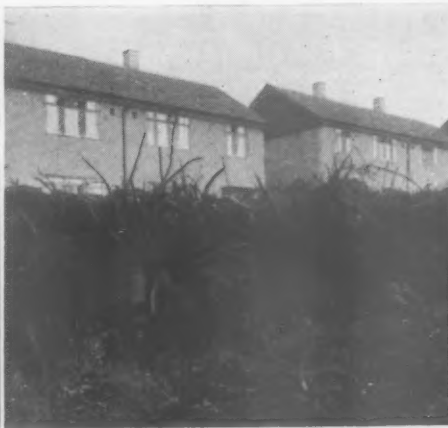
The new alignment appears. . . .
