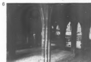
6, vestibule to the chapter house at Chester, late thirteenth century, the earliest English case of piers without capitals supporting the vault.
