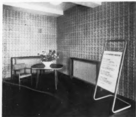
11, wall radiators at Cavendish House, Norwich, made by Gulf Radiators.
