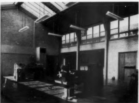
19, the engineering machine shop ; reinforced concrete frame is painted in light terra-cotta.
