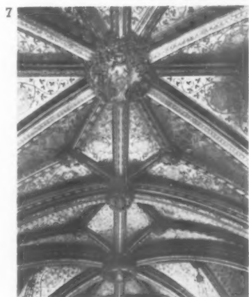
7, lower chapel of the Chapel of St. Stephen at Westminster Palace, now within the Houses of Parliament, begun in 1292, showing the earliest existing lierne vaults.
