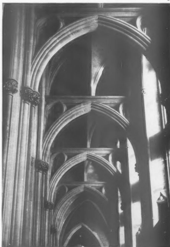
7, lower chapel of the Chapel of St. Stephen at Westminster Palace, now within the Houses of Parliament, begun in 1292, showing the earliest existing lierne vaults.
