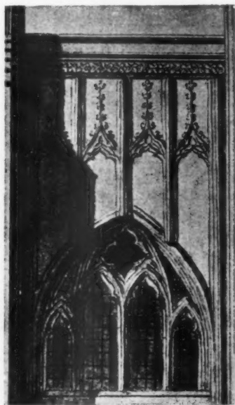
31, the window of the lower chapel of St. Stephen's with descending mullions.
