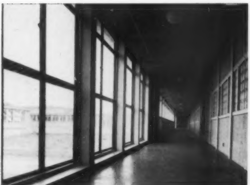
15, typical classroom corridor ; glass brick panels on the right give additional light to classrooms.
