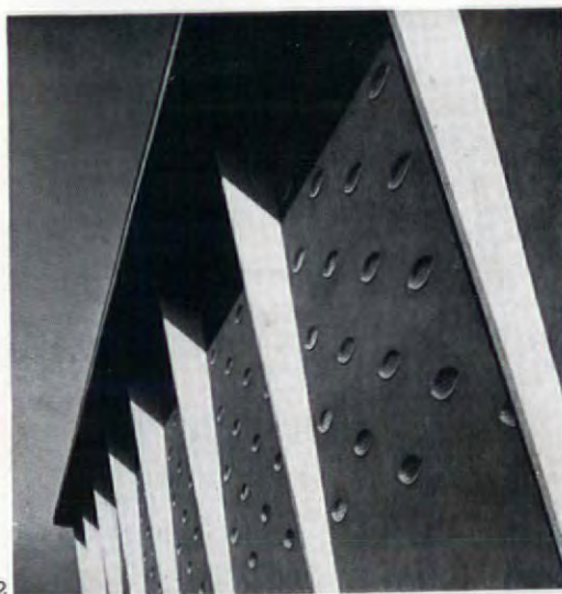
2, the south-west facade of the Lion and the Unicorn pavilion, designed by R. Y. Goodden and R. D. Russell. The eye-shaped windows are intended to provide a pattern of sunlight inside the building, and the louvres conceal the view of Hungerford Bridge. 3, the interior of the Lion and the Unicorn pavilion. The birds have been released from their cage by the lion and the unicorn—twin symbols of British character and tradition. On the end wall is a mural by Edward Bawden depicting English country life.
