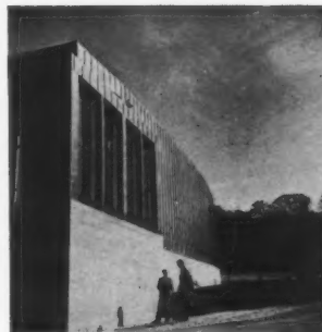
4. corner of the auditorium block.
