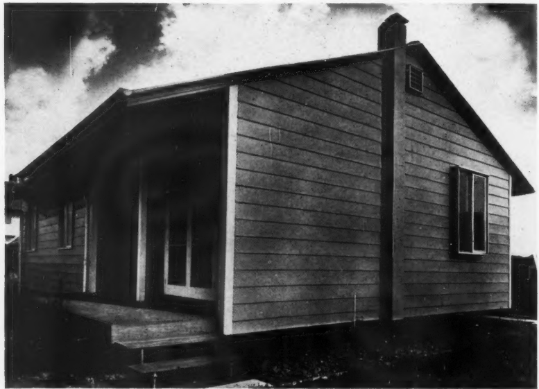
2, general view of the prototype aluminium prefabricated house.
