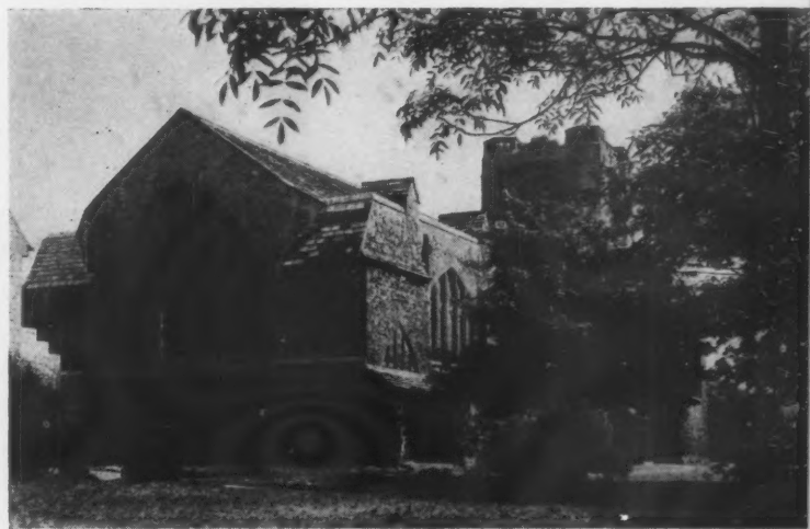
22, general view of the west end of St. Andrew's.
