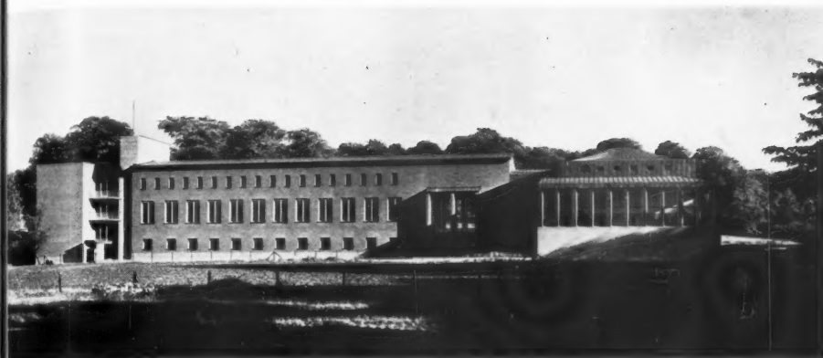
8, the northern façade ; the tall windows on this side of the auditorium provide lighting for the reading space of the library, which lies under the slope of the auditorium floor. 9, the main entrance on the south is at first-floor level and the hall commands a view of the Cathedral through windows over the ground floor entrance on the north.
