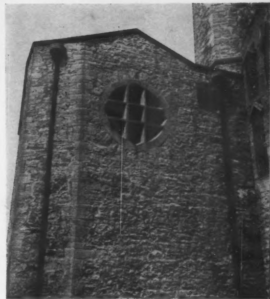
21, the east wall of the Lady Chapel of St. Andrew's. Here, in chastened form, Prior's love of texture still finds expression.
