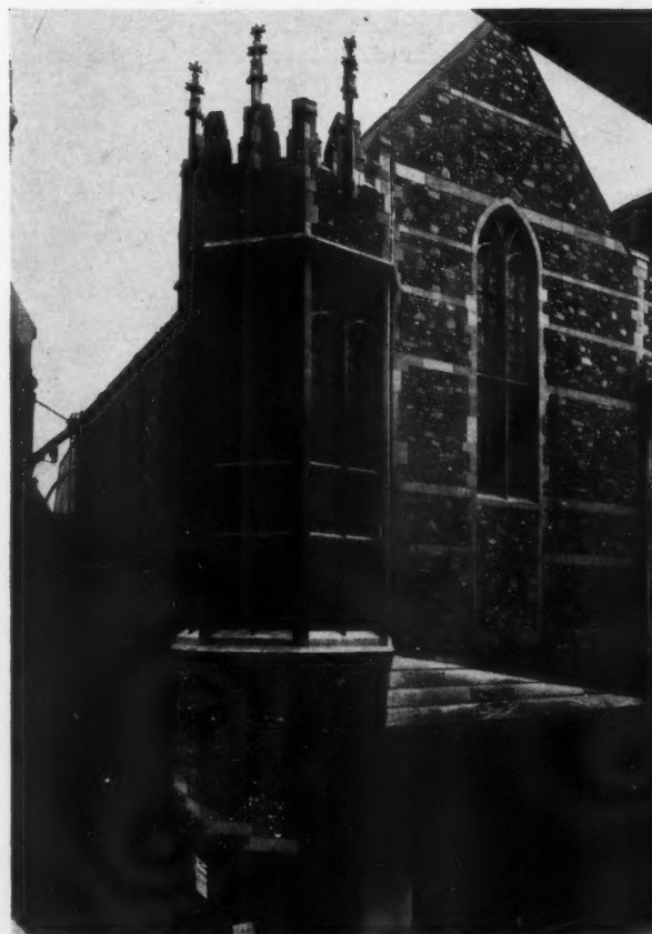
7, the stair-turret of Henry Martyn Hall , Cambridge, 1884–6, with the ends of the tread slabs revealed on the outside of the building.
