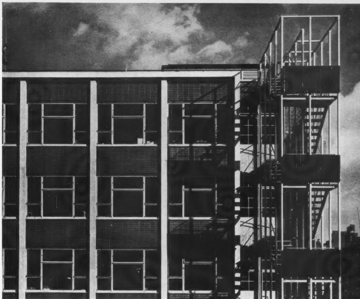
4, part of the new west elevation.
