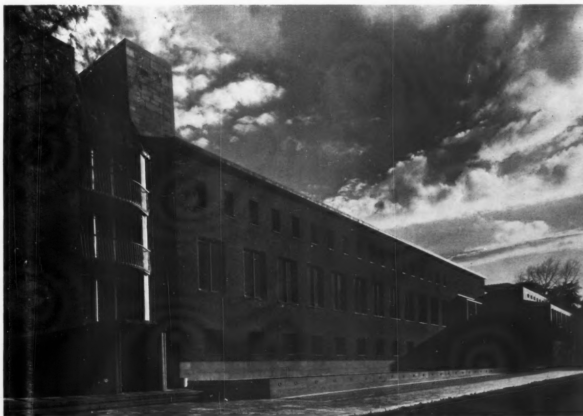
5. view along the northern façade toward the subsidiary entrance. At the extreme left is the entrance and stairwell windows of the office block.
