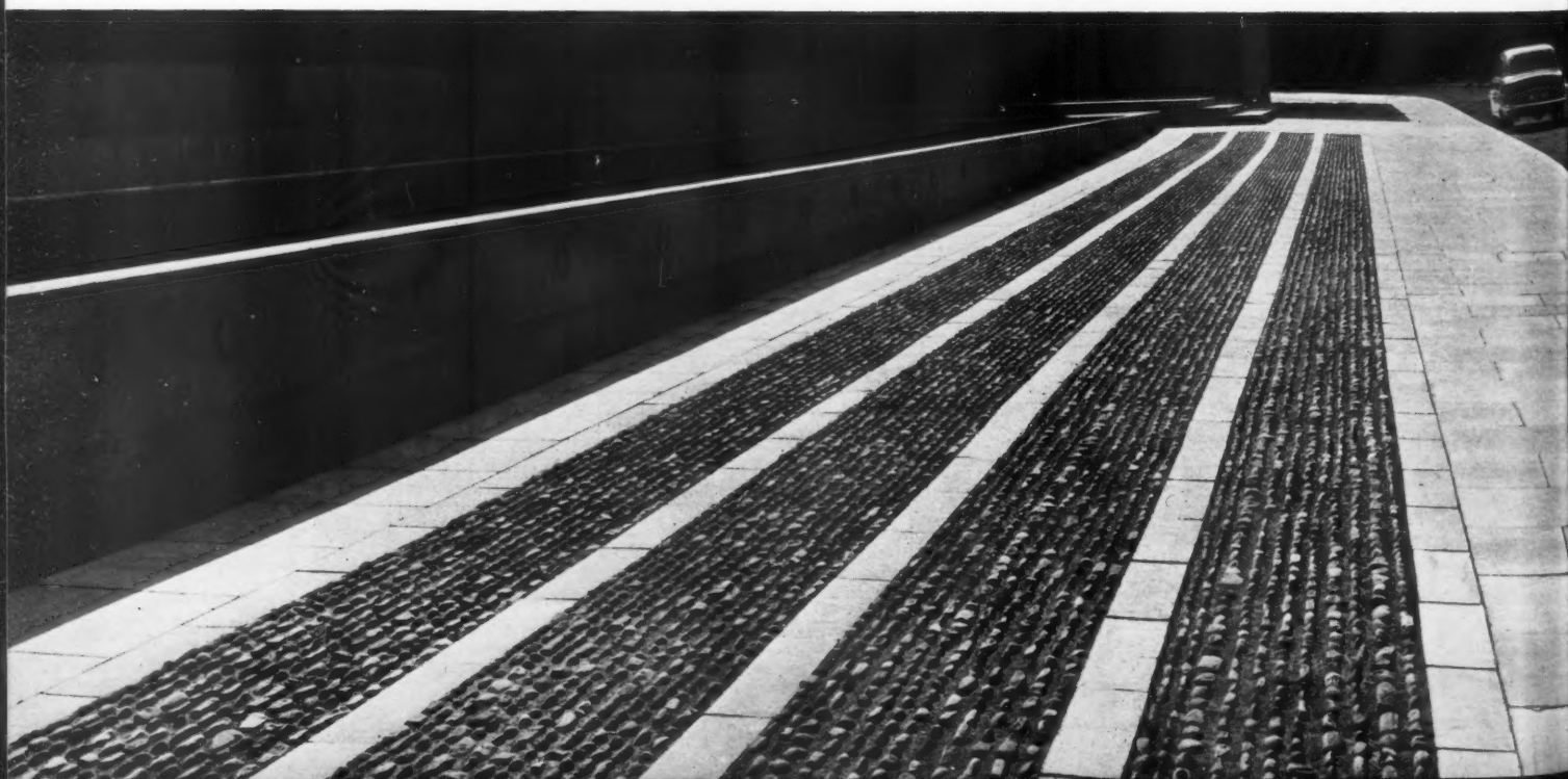
7, cobbles, used on the approach along the northern side of the building, providing textural interest combined with ease of maintenance.
