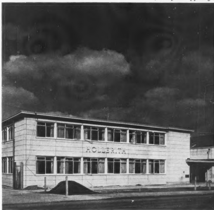
1, south facade of factory 9.
