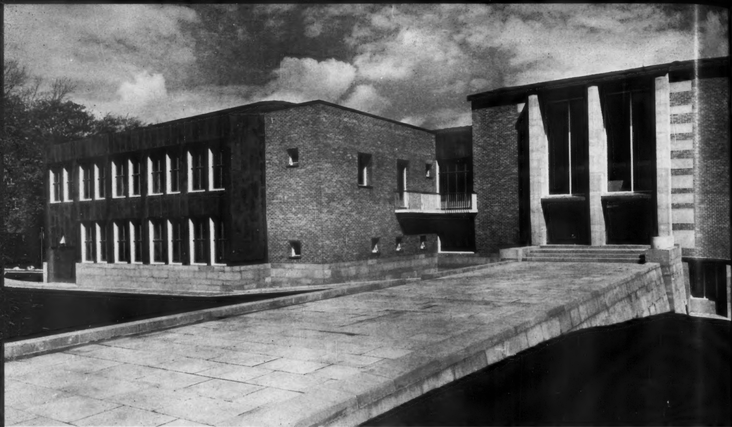
3, the main entrance and auditorium from the south. The panelled surface of the auditorium is of vertical copper sheathing.
