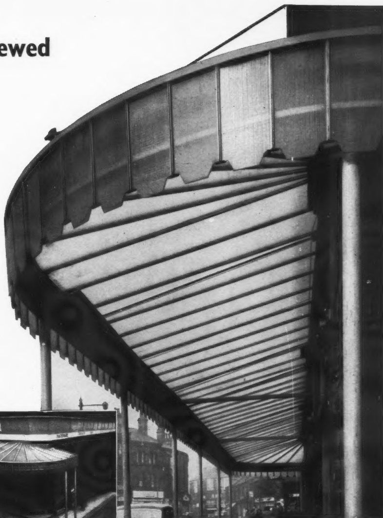
★ Patent Glazing for the New Verandah at Bailey Co-operative Society Ltd.
