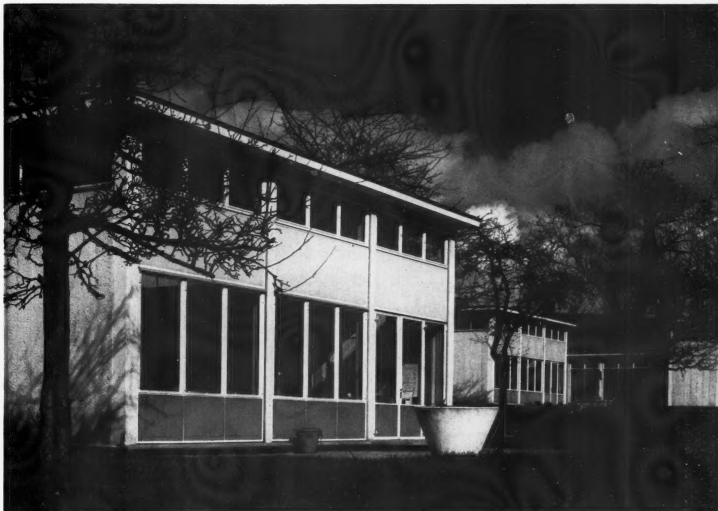
1. from the south, showing three classrooms, each of which is designed as an independent pavilion.
