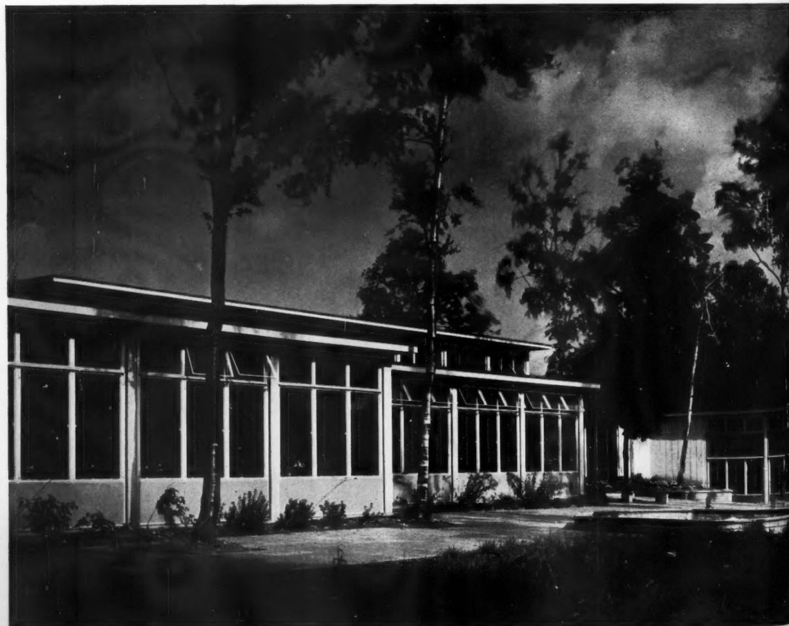
8, infants' classrooms looking on to a tree-planted courtyard. In the background on the right is the dining-room-kitchen wing. Above the roof of the classrooms can be seen the upper part of the assembly hall.
