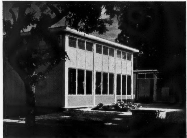
Aboyne Lodge Infants' School, St. Albans. C. H. Aslin, C.B.E., F.R.I.B.A., County Architect.
