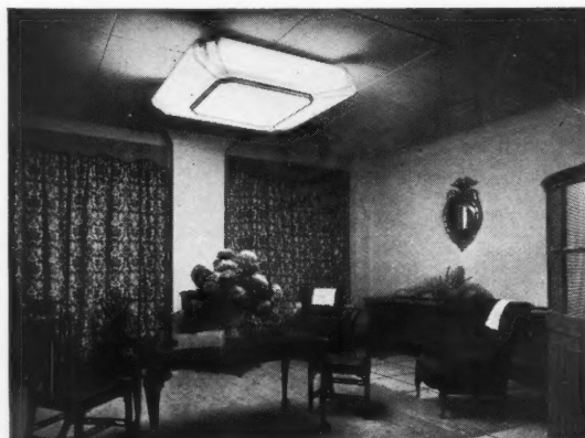
A multiple installation at the Banker's Clearing House, London. The unusual single-rod suspension fittings carry ATLAS FM/2080 fluorescent units. Contractors: Messrs. Grierson, Ltd.
