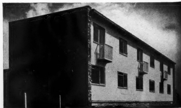
4, south and west facades of terrace house block.
