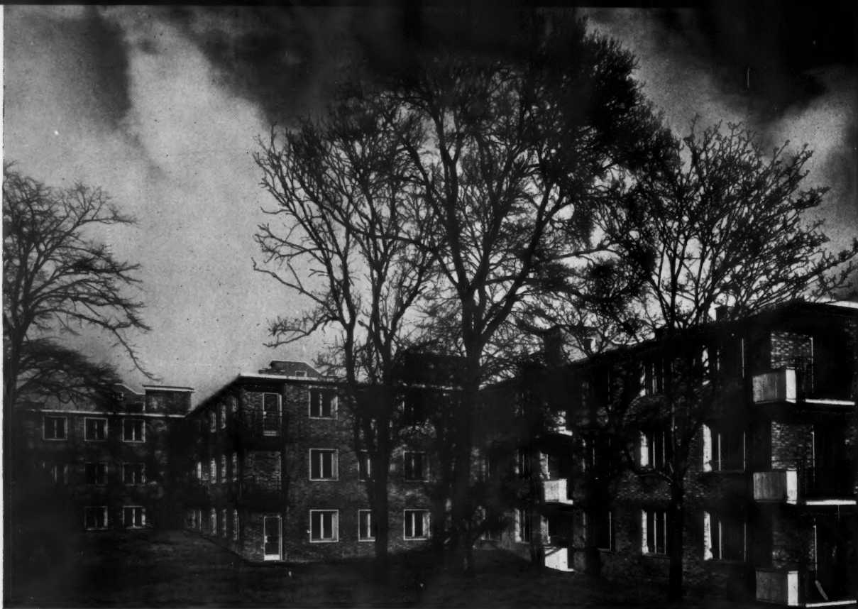
Looking north at the staggered three-storey block.
