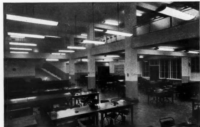
A multiple installation at the Banker's Clearing House, London. The unusual single-rod suspension fittings carry ATLAS FM/2080 fluorescent units. Contractors: Messrs. Grierson, Ltd.
