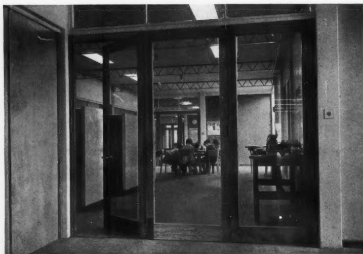
*Templewood C.P. School, Welwyn Garden City. Sliding, folding partitions (glass and flush), chalkboards and furniture.
