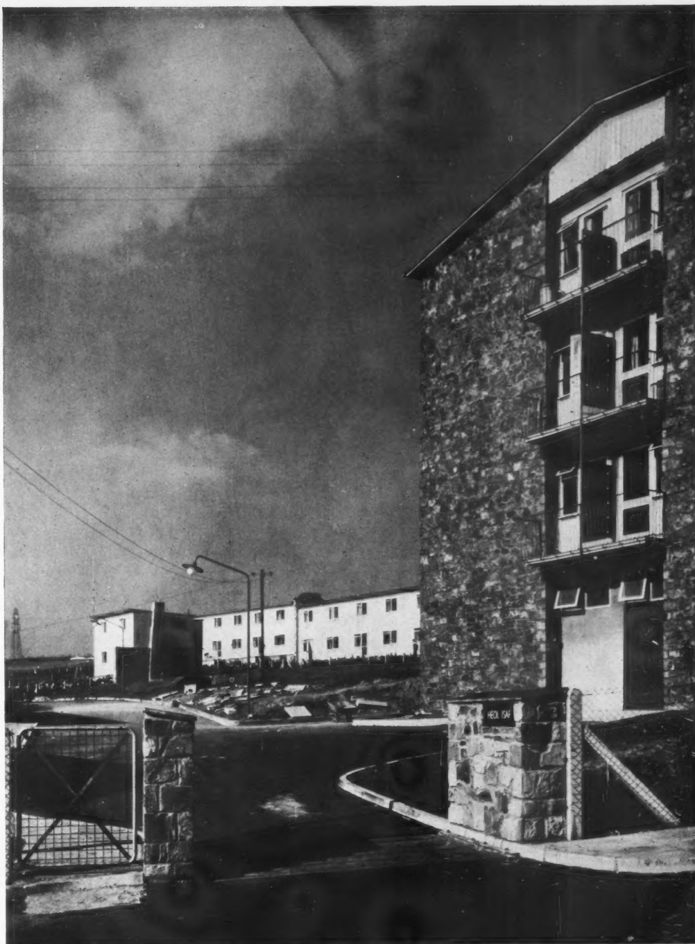
Looking north-west with the south facade of a three-storey block on the right.
