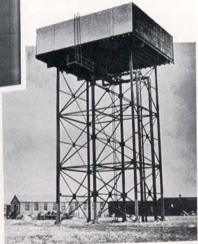
Below : An "airborne" Mather & Platt tank of 80,000 gallons capacity on active service with the R.A.F.
