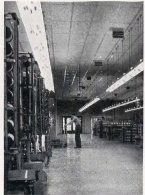
In the ring-doubler section of the Brocklehurst Yarns factory near Cardiff, the continuous rows of ATLAS FE/0081 lighting units are protected by the "Miracoat" finish against the moist atmosphere prevalent in Spinning Rooms.
