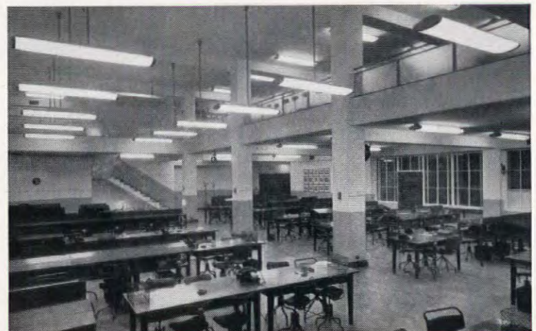
A multiple installation at the Banker's Clearing House, London. The unusual single-rod suspension fittings carry ATLAS FM/2080 fluorescent units. Contractors: Messrs. Grierson, Ltd.
