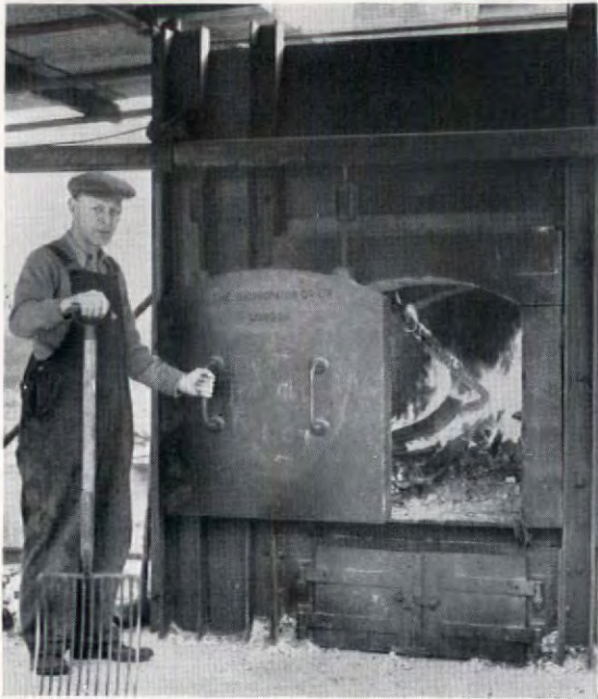
Above: Incinerator installed at a film studio to destroy general waste, film sets and scenery.
