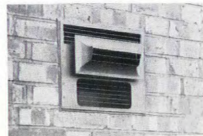
The terminal can be fitted even in proximity to overhanging, or other projections. There is no flue pipe or cowl.
