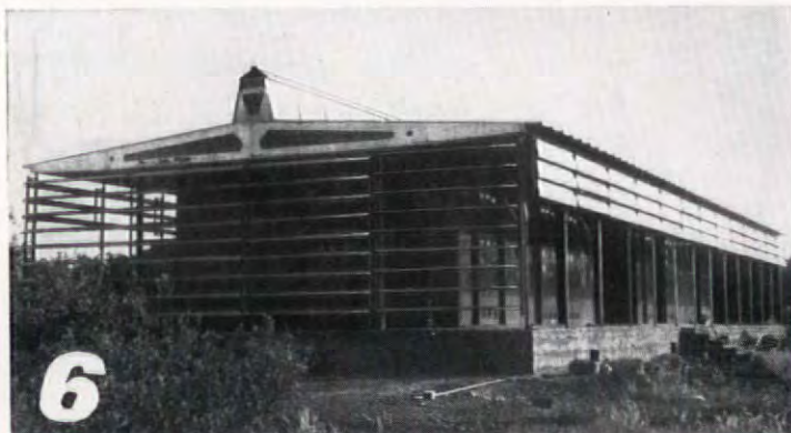
1 , assembly of tie beams on the prepared concrete foundation; 2 , erection of portal frames and sectional roofing beam; 3 , portal frames and roofing beam completed; 4 , assembly of roofing and wall panels; 5 , panelling completely assembled and gable beam in position; 6 , the adding of the brise-soleil; 7 , the completed house.
