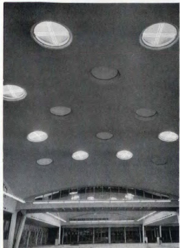
Interior night view of one of the nine domes showing the general layout of the daylight and fluorescent portlights, and the fluorescent troughing which simulates the daylight from the vertical glazing just above it.
