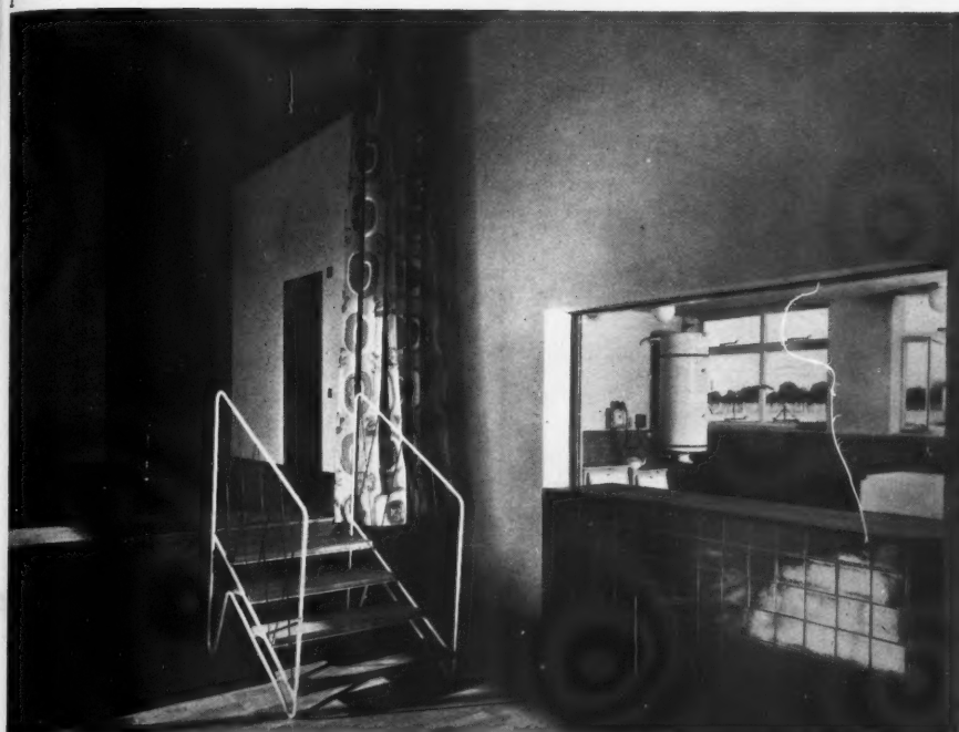
7, part of the stage in the assembly hall and the kitchen hatch. The steps are of welded steel with hardwood treads, and slide along the front of the stage.
