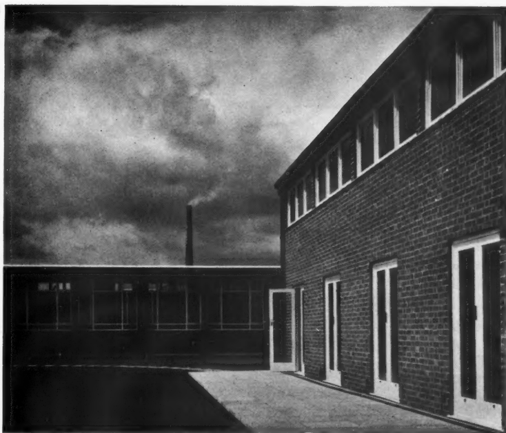
Looking west with the south wall of the conference room on the right.
