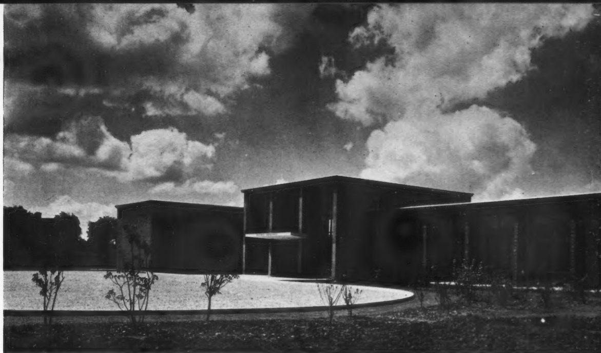
The east facade looking south-west.
