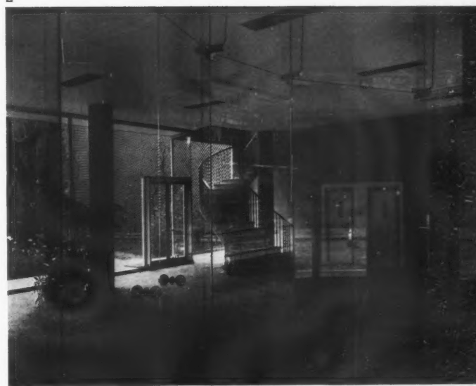
1, the façade of the new office block seen from Rue La Pérouse. 2, the armour plate glass doors between the public lobby and the main hall of the office block. The helical staircase which rises round a column is free standing between floors.
