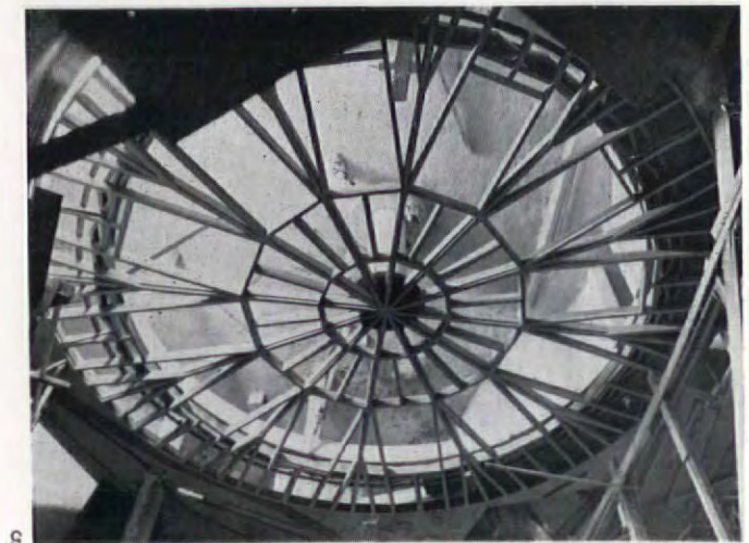
5 is the wooden structure of the revolving stage photographed during construction. 6, a general view of the auditorium.
