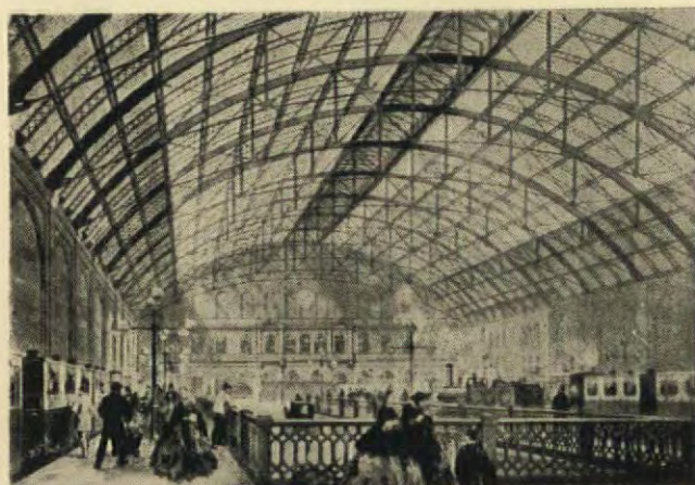
London, Charing Cross Station, 1862-64, E. M. Barry, arch., J. Hawkshaw, eng., span 170 ft.
