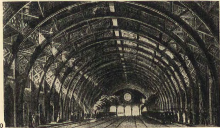
10 Munich, Hauptbahnhof, 1847-49, F. Bürklein, span 80 ft., wooden arches.
