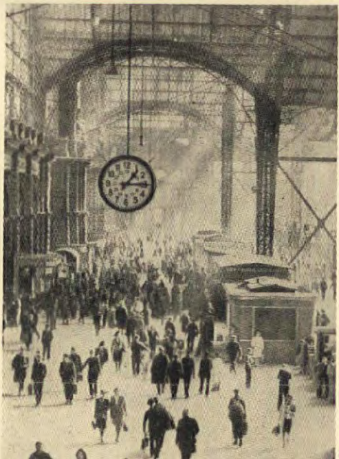
20 Frankfurt-am-Main, Hauptbahnhof, 1879-88, J. P. H. Eggert, three arched spans 183 ft. each.
