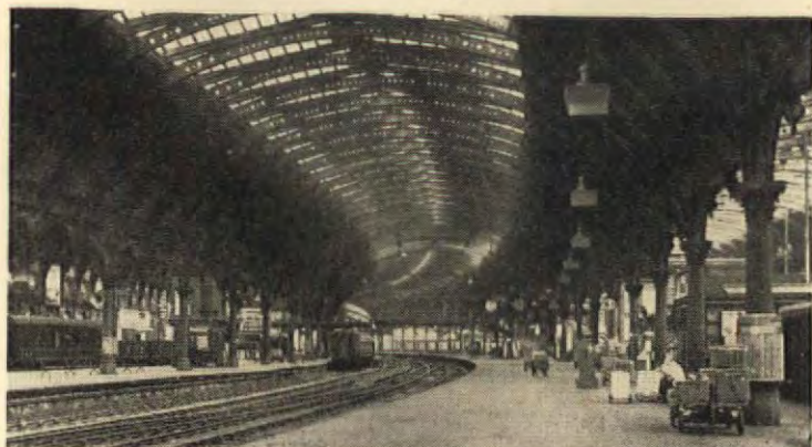
19 Philadelphia, second station, 1871-77, by T. Prosser, B. Burley and W. Peachy, wrought iron arches, widest span 81 ft.
