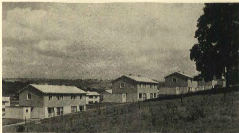
a Houses at Bath designed by Frederick Gibberd. This type was evolved by the British Iron and Steel Federation: examples here have cavity walls with ground floor rendered and first floor faced with vertically hung metal sheathing.
