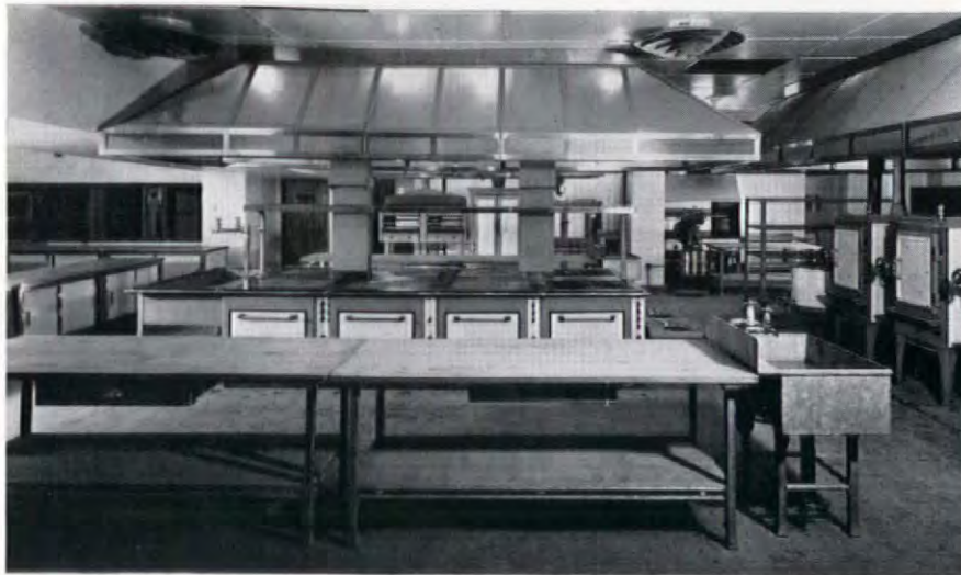
A general view of the all-gas kitchen which will cater for 1,800 people at three sittings. Cooking apparatus was manufactured by Benham, the company also planned and installed the kitchen.
