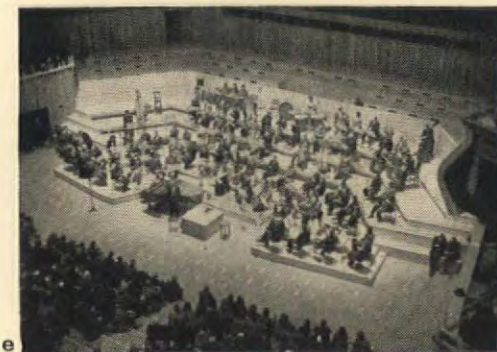
The first music played in the auditorium was at a tuning test which took place on February 14, 1951. e, the orchestra platform during this test. f (below), three alternative arrangements of the platform, which is adjustable to suit different orchestral layouts. The arrangement on the right is that shown in the photograph.
