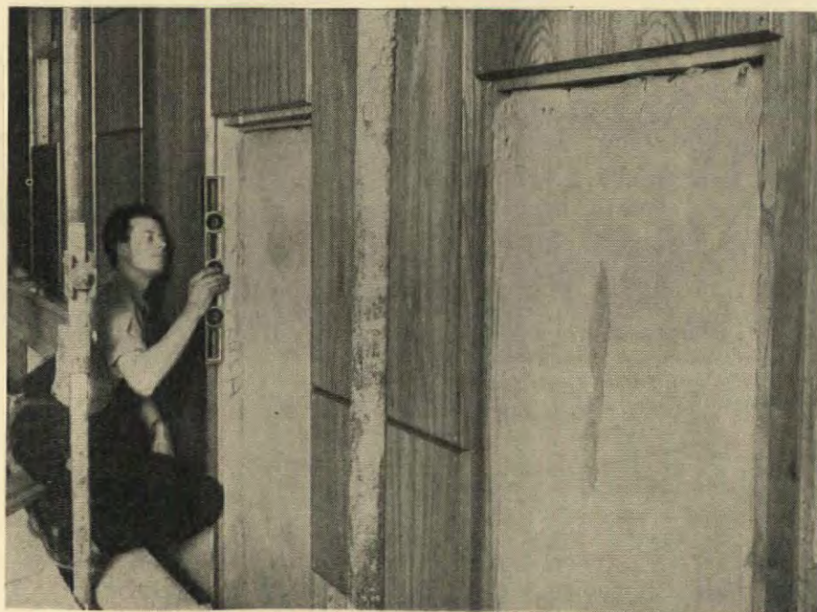
g, wall panelling at side of auditorium, with panels removed to show rock-wool filling.
