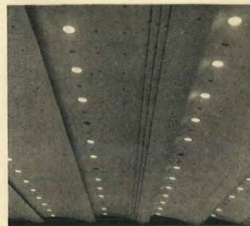
h, the ceiling, showing the plugged holes for Helmholtz resonators to be inserted later if necessary.
