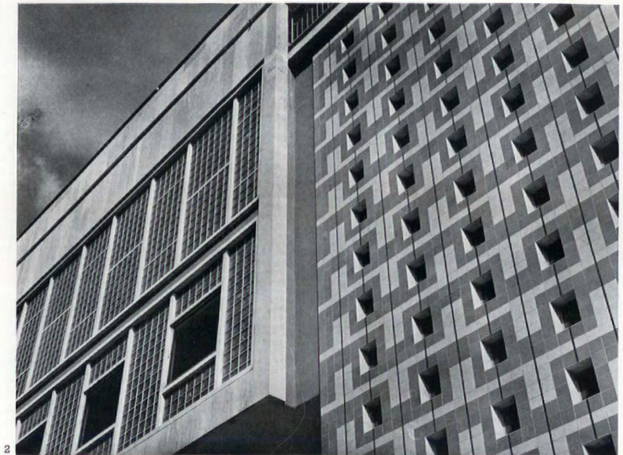
2, looking up at the Hungerford Bridge side of the building. On the left are the glass lens windows, in a frame of Portland stone, that light the side promenades and bars at mid-stalls and upper stalls level. On the right are the small windows of the rear staircases. The wall surface is of pale blue and white tiles.
