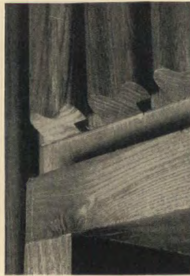
'Copenhagen ribbing,' a type of wood wall-surfacing devised for its absorbent properties. i, the panelling partly in place, with the rock-wool filling behind. j, a detail of Copenhagen ribbing showing the slits between ribs. k, the surface texture given by the Copenhagen treatment. l (below), absorbents at the back of the auditorium take the form of padded leather panelling with air spaces and rock-wool behind.
