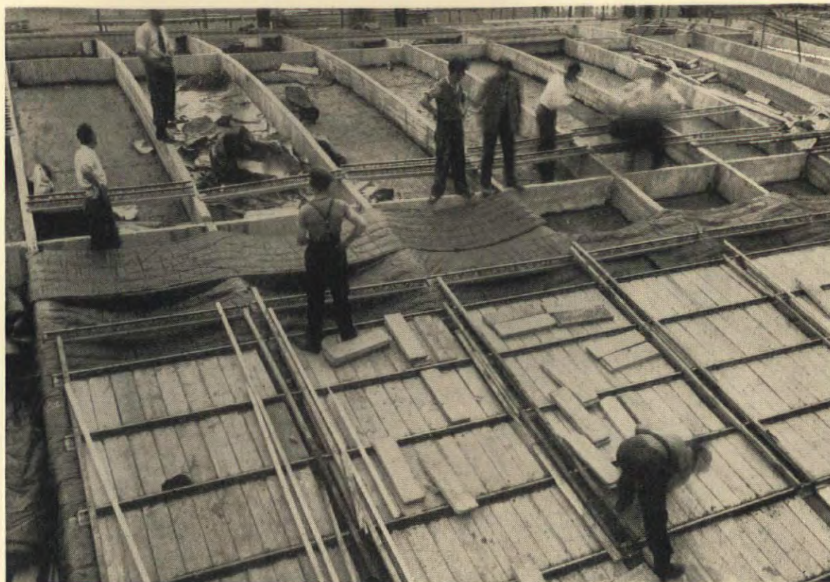
o, the roof under construction; the outer concrete skin rests on insulating blankets of glass-wool over sleeper walls carried by the inner skin.
