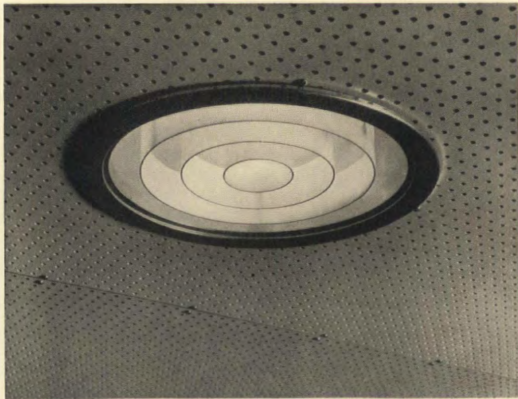
p, perforated plastic panels as used in the ceilings of the foyers, shown surrounding one of the light fittings. Behind the panels is an air space partly filled with rock-wool. q (right), perforated metal covers for the absorbent around the edges of the doors, to keep noise from going through the cracks.
