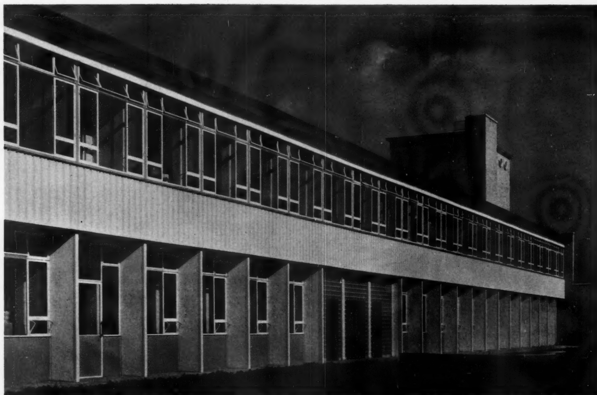
Classroom wings from the south-west.
