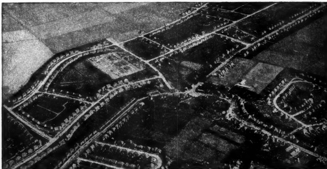
Peterborough Corporation Housing Scheme, Peterborough, Northants.
