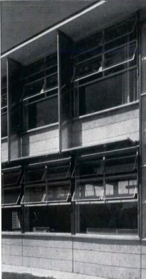
**Windows with fins** Streamlined aluminium sunshields, deflectors and cills (left) specially designed for the building by Williams & Williams form part of the windows of the special subject classrooms in the main block. The vertical fins are 12 ft. high and project 1 ft. 9 ins. The horizontal deflectors which shield the ground floor windows from overhead sunshine are pivoted to raise and lower for ease of cleaning.
