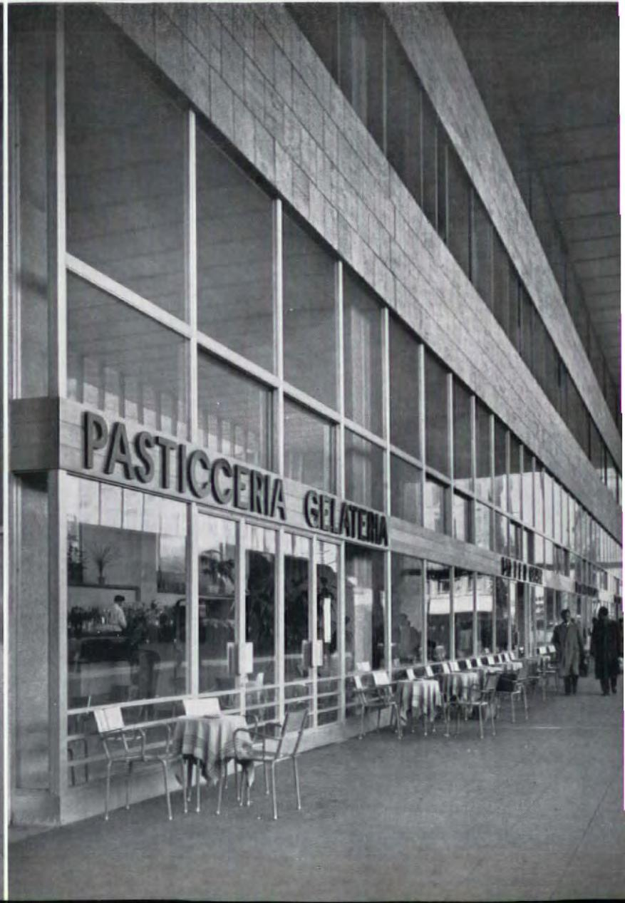
tween the Via Giolitti and the Via Marsala. The upper part of the wall over the platforms is of light metal framing glass panels.
