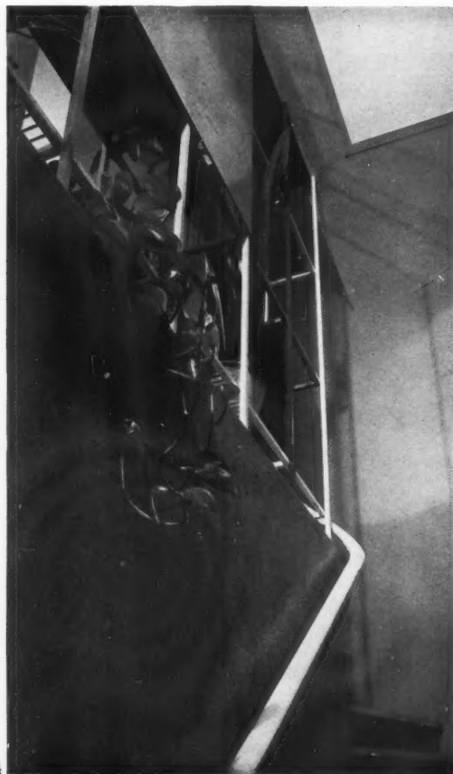
The head of the staircase leading to the auditorium in the basement. The side wall is of black Tinos marble.
