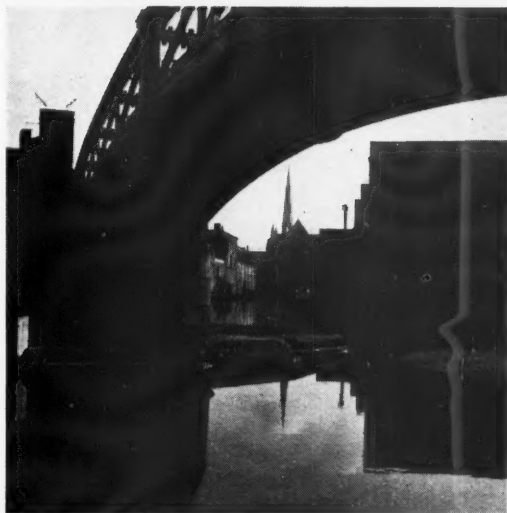
three views of the Birmingham canal
