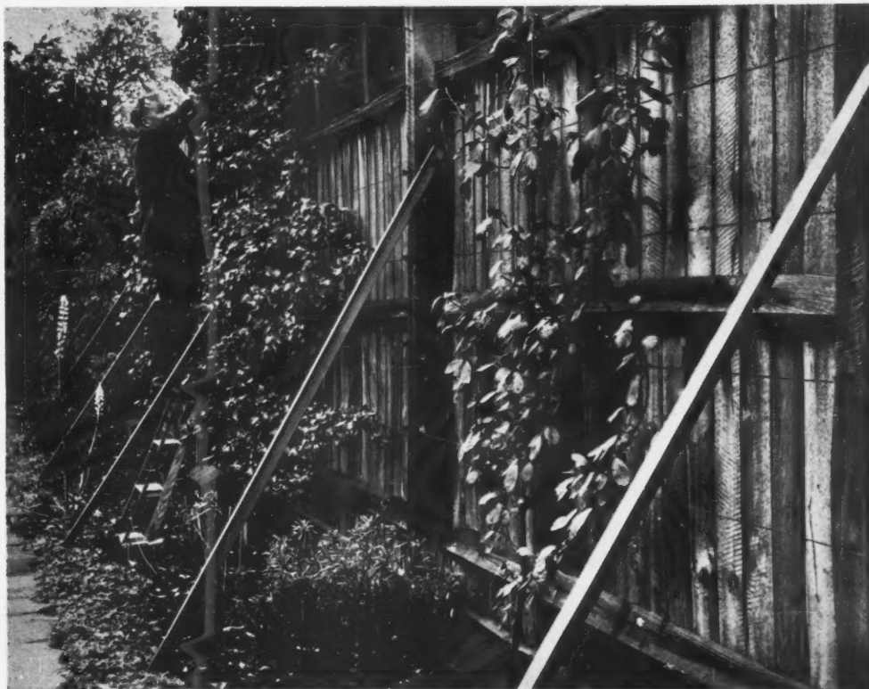
THIS FRUIT FENCE, 3 MILES FROM THE CENTRE OF BIRMINGHAM, HAS 17 GALVANIZED STEEL STRUTS, FIXED IN 1920. THEY WERE FIRST PAINTED IN 1949; THERE WAS NO CORROSION
