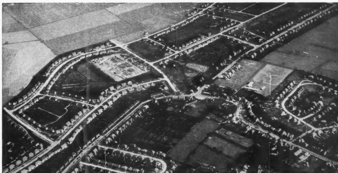
Peterborough Corporation Housing Scheme, Peterborough, Northants.
