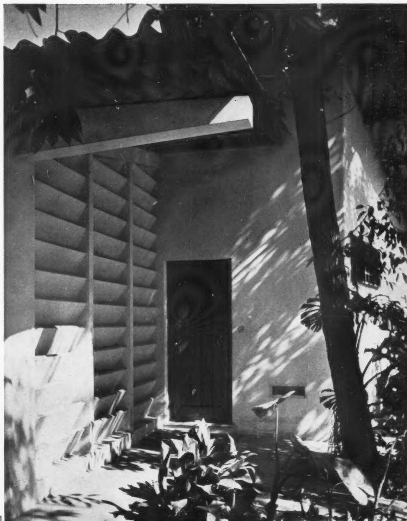
1 the front door. The louvres are of reinforced concrete and are placed to protect the dining room from the prevailing wind
