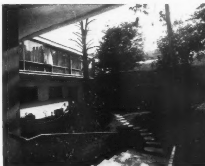
14 the courtyard garden, with the pathway leading to the annex (block 7).
