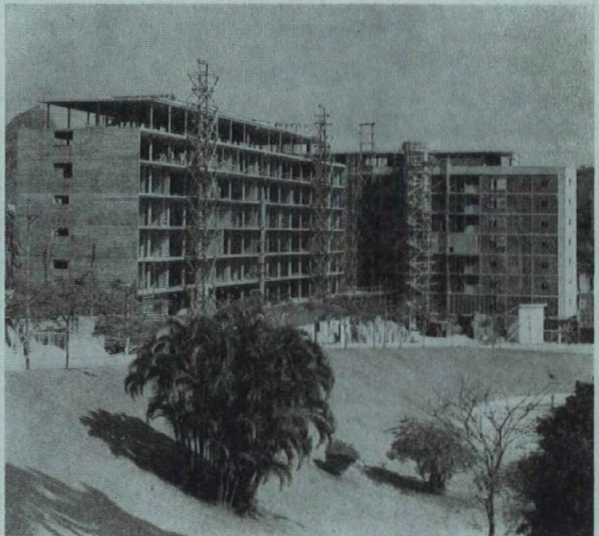
4, the first two blocks, "Bristol" and "Nova Cintra", photographed while still being built, to show the reinforced concrete slab and column construction.
