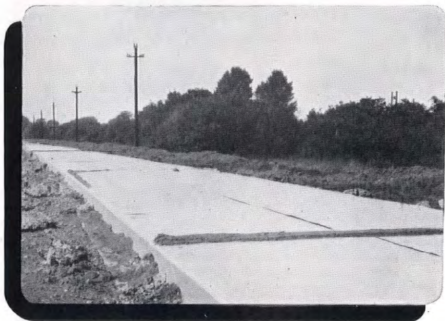
Typical example of a concrete road slab blanketed with Sisalkraft.
