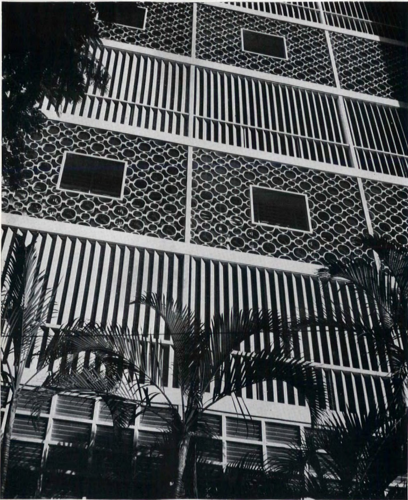
7. close-up of part of the façade of "Nova Cintra" showing the vertical brise-soleil and open ceramic grilles on alternate floors. The horizontal brise-soleil in small panels at the foot of the picture light the upper part of the ground-floor shops.
