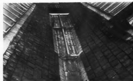
8, super purity aluminium used for valley gutter lining.
