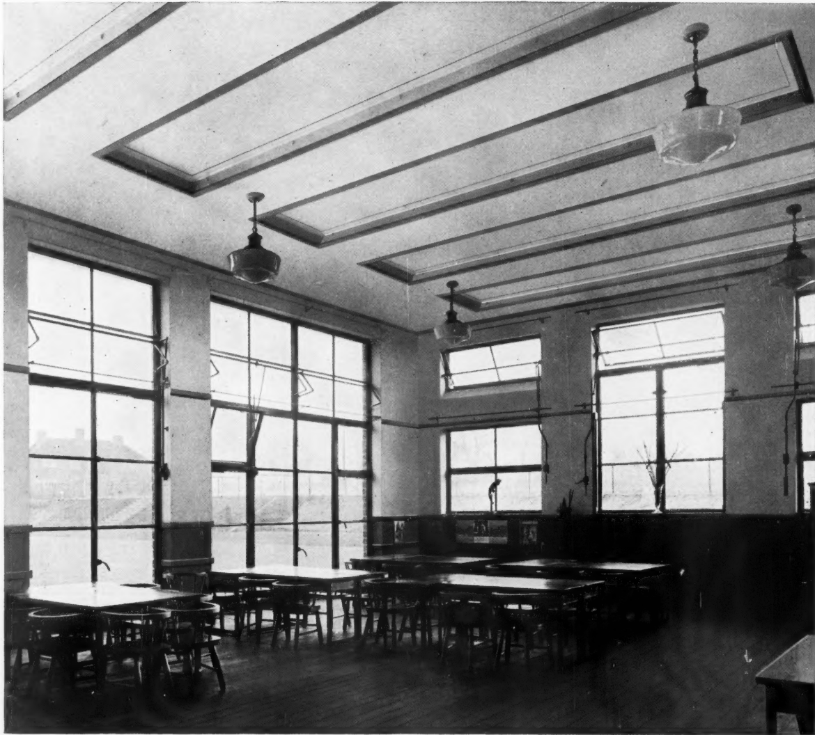
The Ideal Rayrads illustrated are recessed about 3 inches in the ceiling and are included in the decorative scheme.
