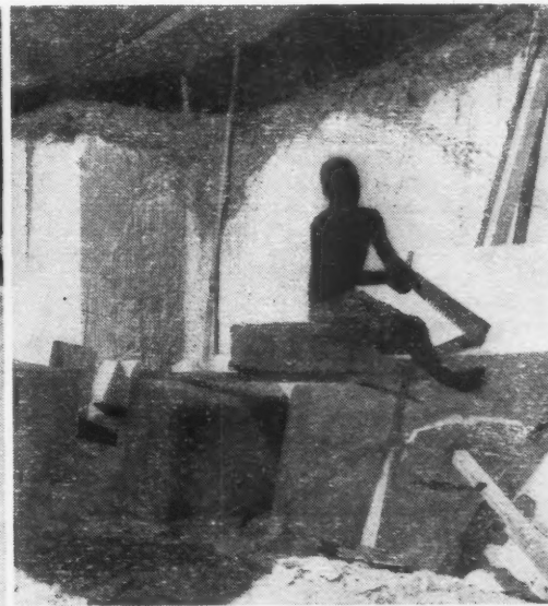
Early settlers coming from the West Country and the Cotswolds found that the local stone, though soft enough to be cut with a handsaw, hardened on exposure to the atmosphere. Owing to its porous nature, however, it was necessary to render it.
