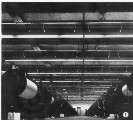
1 A recent installation, providing an average illumination of 40 lumens per sq. ft. in a silk weaving shed of Messrs. Tootal, Broadhurst, Lee & Co. Ltd. The shed measures 229' x 96' 8".
