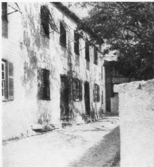
Early settlers coming from the West Country and the Cotswolds found that the local stone, though soft enough to be cut with a handsaw, hardened on exposure to the atmosphere. Owing to its porous nature, however, it was necessary to render it.
