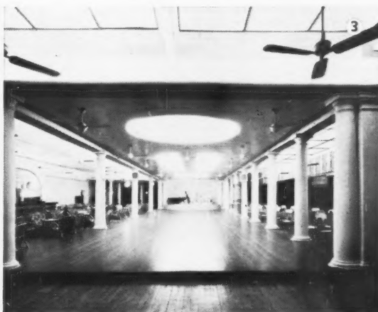
3 This Ballroom of the Selangor Club, Kuala Lumpur, Malaya is lighted by ATLAS Peach 3 ft. 30 watt lamps, the covers being specially designed for this installation.
