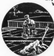
Roof and Floor Screeds.
