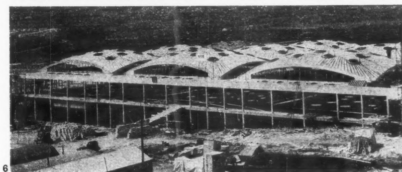
4, 5 and 6 are typical examples of shell construction. The Factory Canteen in Essex, by Edward Mills, 4, shows the architectural treatment of a cylindrical shell; the special effect being achieved by cantilevering out only the actual roof, stopping the beams short so that only part of the construction is visible from the outside. The locomotive sheds at Chalons-sur-Marne, 5, is one of the largest shell constructions of this type carried out recently. 6, a factory at Brynmawr by The Architects' Co-operative Partnership, makes the most extensive use of domes of any building in this country. The domes are designed on a rectangle, and the spandrels are used for lighting purposes.
