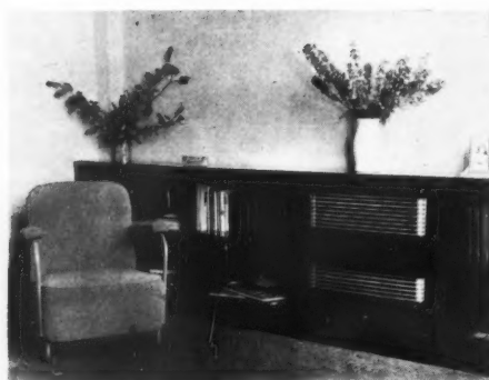
15, the inset Thermovent electric space heater.
