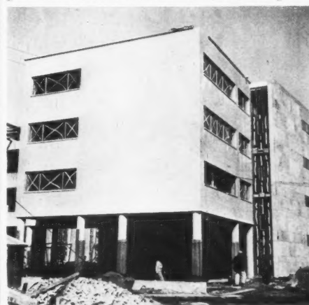
8, progress photograph of the new graduate centre, Harvard.
