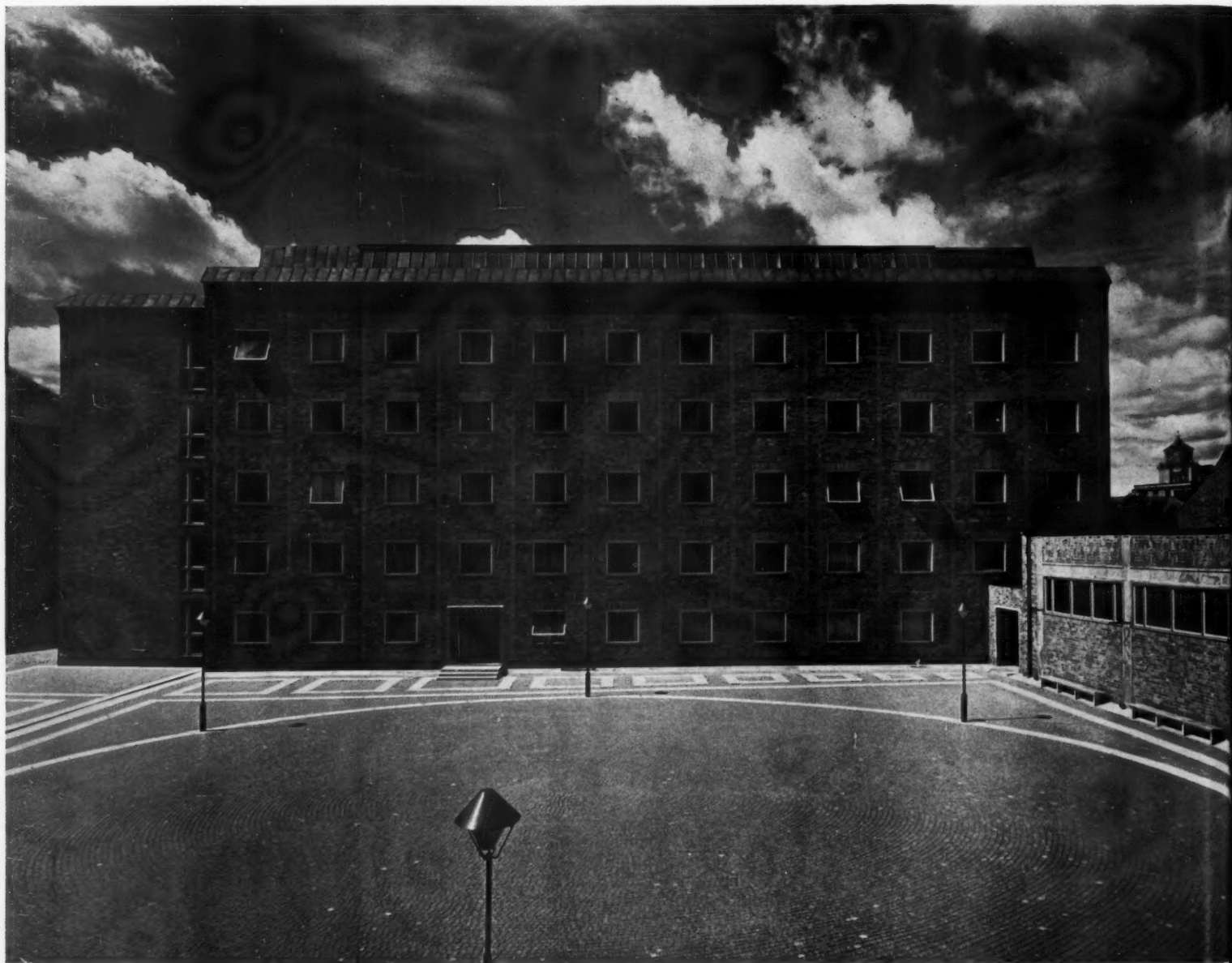
2, looking from the east across the main court to the drawing office building. The courtyard is paved with stone setts laid concentrically
