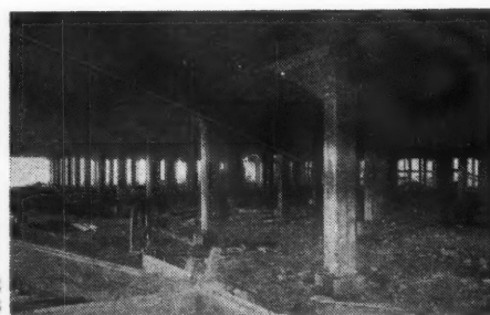
2, Store building at Bristol for Messrs. E. S. and A. Robinson. This building, which was erected in 1939, is a typical flat slab construction, designed in accordance with the Code of Practice. Sizes of column heads and drops are governed by the regulations, leaving the designer to arrange the spacing of the columns, and their size, depending on the load. Although the Grain Elevator at Kansas City, 3, shows no new departure in construction it does emphasize the potential beauty of concrete employed entirely functionally on a large scale.
