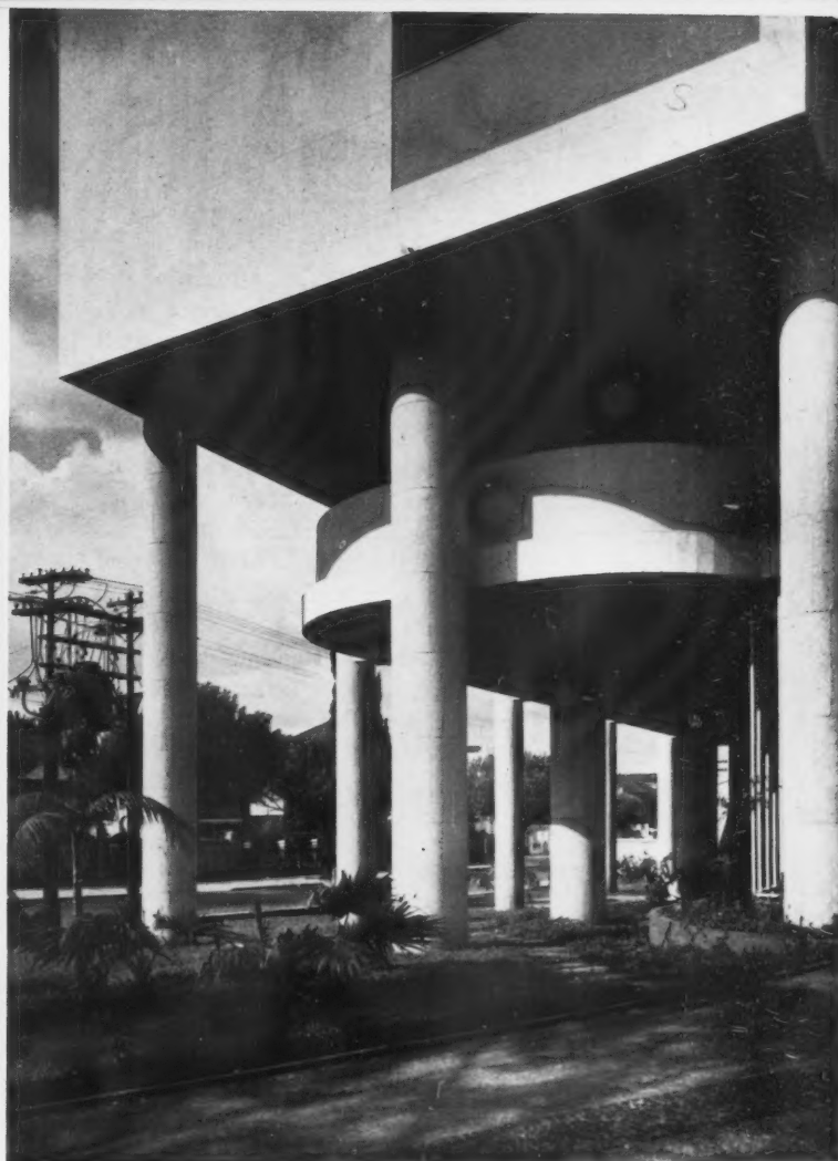
18, 19, two ground floor details, showing the effect of raising the whole block on columns and taking the garden beneath it. On the left is the arcade of shops. 20, a general exterior
