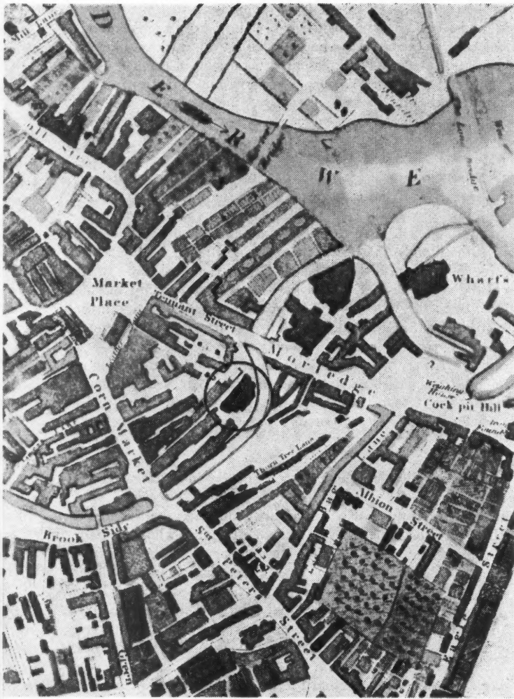
Part of Derby from the Rogerson map (1819). The circle marks William Strutt's Calico Mill, 1792-93, the first multi-storeyed iron-framed incombustible building. It inspired English 'fireproof' mill construction and led directly to the steel skeletons of modern skyscrapers. (Courtesy of Dr. W. Alfred Richardson.)
