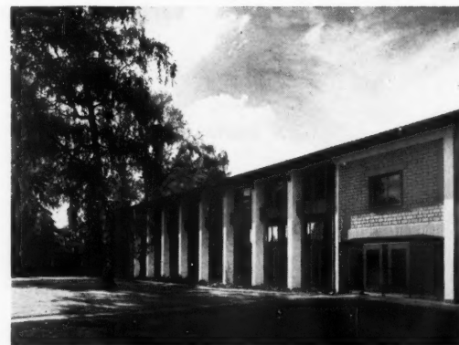
3, the gymnasium showing the windows and double-doors of unsplinterable glass. Window frames are of varnished wood
