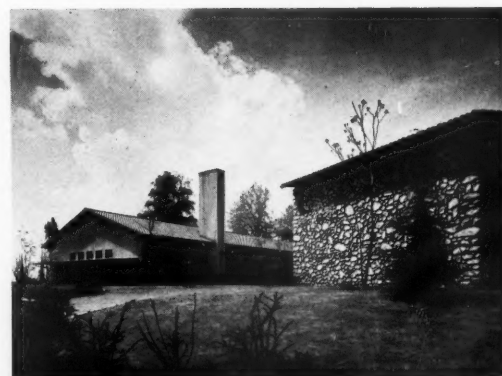
4, the main entrance to the school with the gymnasium block in the background and the end wall of the music room in the foreground
