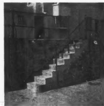
The steps are good, but ill-conceived railings destroy their simplicity.
