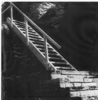
When the flight of steps has to be poised in mid-air, as on the diving board, 136, or the ladder-form of 137, a railing is essential for safety, but the minimum safeguard is sufficient.
