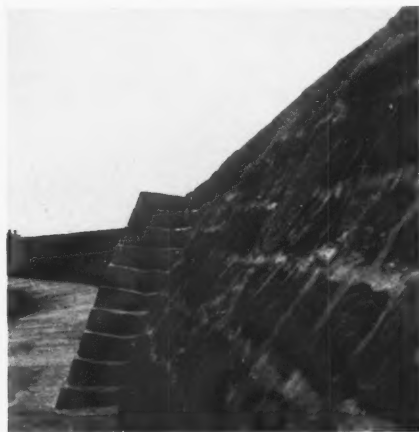
The steps in 134 and 135 are practically part of the wall. The latter is designed most ingeniously to get one safely up a sloping parapet, where a railing would only be a hindrance.
