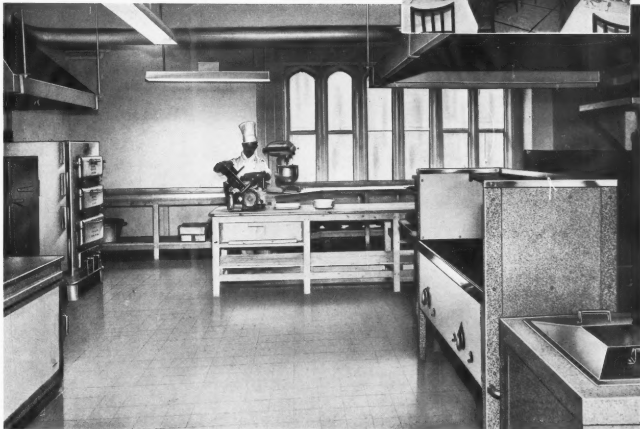
A recent installation in the London Office, Strouger House, Victoria Embankment, for the Automatic Telephone and Electric Co. Ltd. (Architects: Sir John Brown, A. E. Henson and Partners.)
