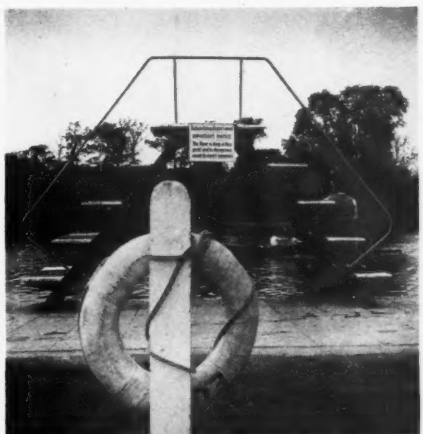
When the flight of steps has to be poised in mid-air, as on the diving board, 136, or the ladder-form of 137, a railing is essential for safety, but the minimum safeguard is sufficient.
