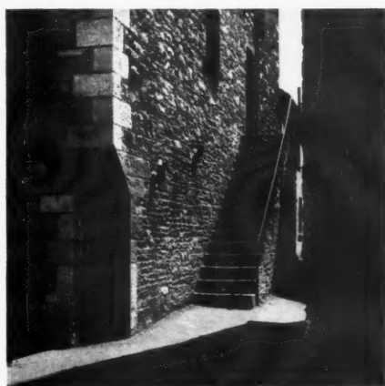
The steps in 134 and 135 are practically part of the wall. The latter is designed most ingeniously to get one safely up a sloping parapet, where a railing would only be a hindrance.
