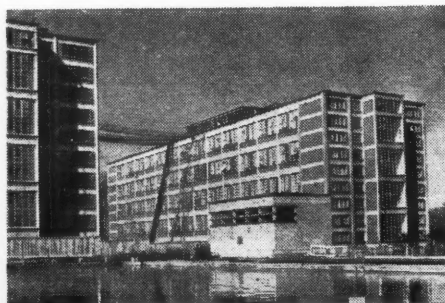
3, new factory building with swimming pool
