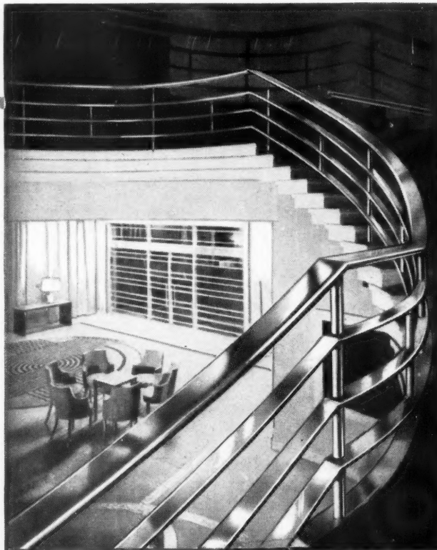
Illustrated shows Entrance Hall, circular staircase with "Birmabright" Handrail and open-type balustrade, at the Midland Hotel, Morecambe.
