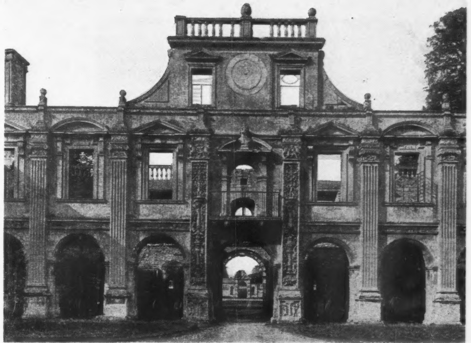
2, the north side of the court of Kirby Hall, Northants, shown by Mr. Summerson to have been built, in all probability, by Thomas Thorpe, John Thorpe's father. The attic storey and window dressings are seventeenth century alterations.
