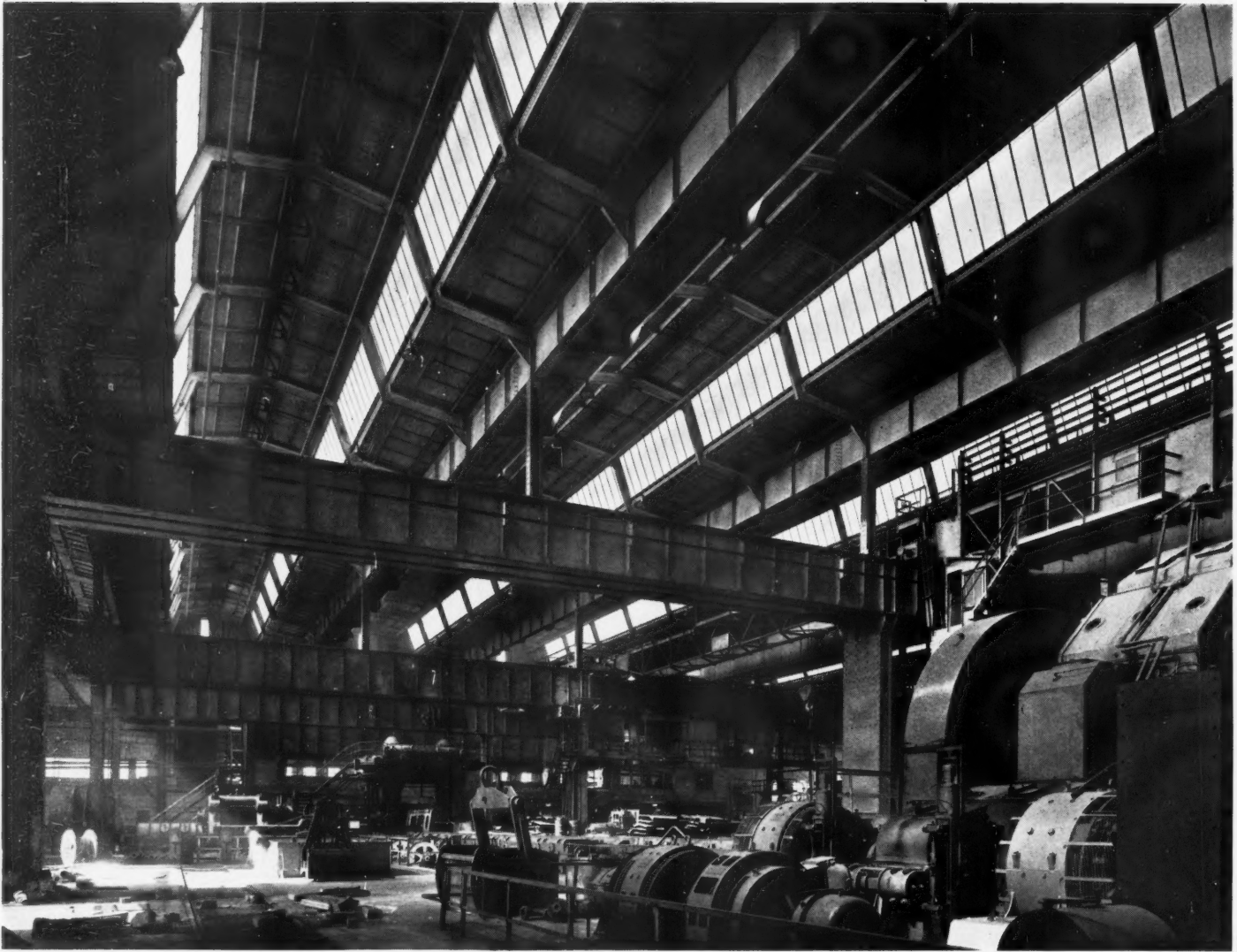
13, interior of the new steel rolling mill, looking towards the control bridge; this gives a clear picture of the roof construction, and illustrates the need for capable site organisation, as the heavy steel rolling machinery shown was in operation while alterations were being made.
