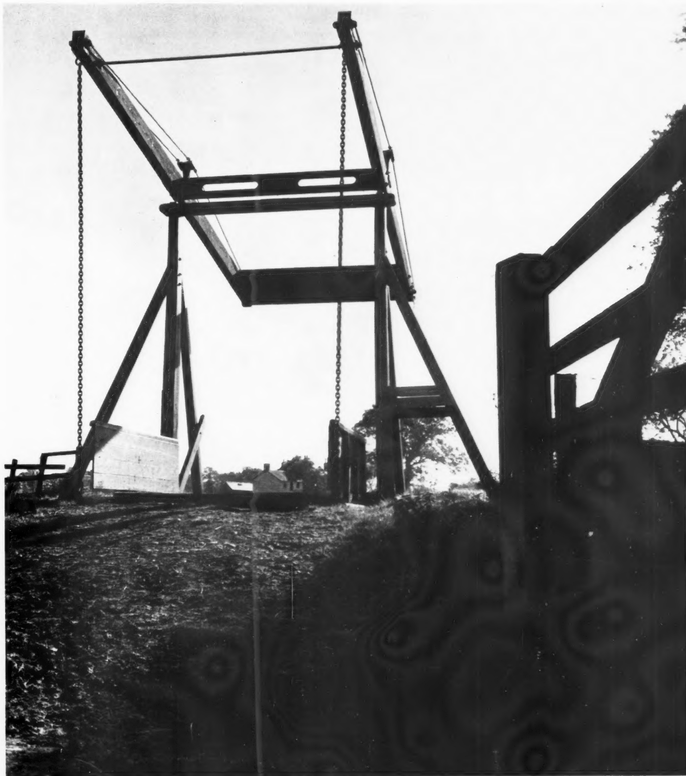
A drawbridge at Whitchurch on the Welsh Section of the Shropshire Union, raised manually by pulling on a chain.
