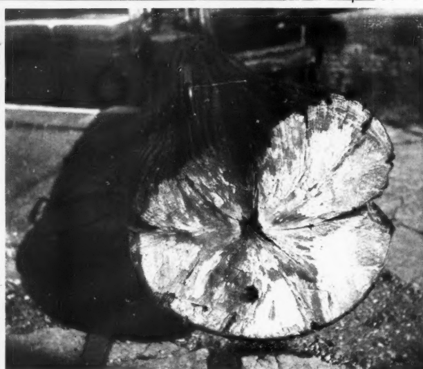
Lock balance beams project from lock gates, balance their weight and act as levers. They are usually of great solid pieces of timber, but new beams are often of steel weighted with concrete. Time gives the timber beams impressive textures. 160, stop-lock at Marston Junction, at the entrance to the Ashby-de-la-Zouch Canal, from the Corentry Canal. 161. 162, two lock beams on the Grand Union.
