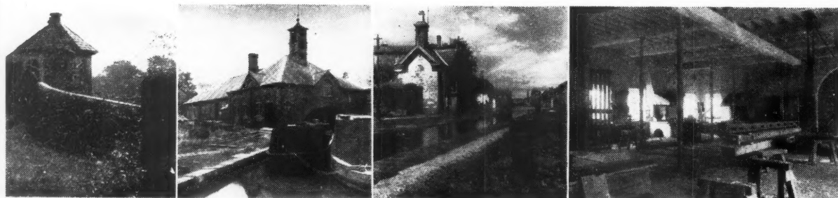
48, octagonal toll-house on the Staffordshire and Worcestershire Canal. 49, maintenance yard on the Coventry Canal. 50, toll-house of 1853 at Stourport. 51, lock repair and building shop with cast-iron pillars at Marsden on the Huddersfield Canal.
