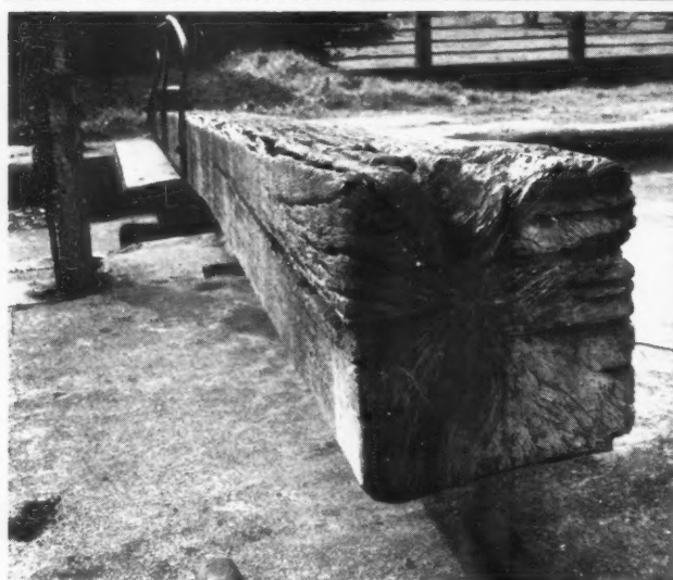
Lock balance beams project from lock gates, balance their weight and act as levers. They are usually of great solid pieces of timber, but new beams are often of steel weighted with concrete. Time gives the timber beams impressive textures. 160, stop-lock at Marston Junction, at the entrance to the Ashby-de-la-Zouch Canal, from the Corentry Canal. 161. 162, two lock beams on the Grand Union.
