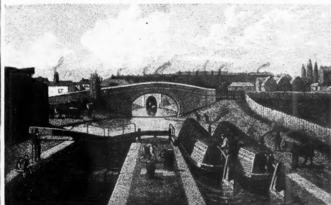
DOUBLE LOCK An engraving of 1827, from a drawing by Thomas Shepherd, of the double lock and east entrance to the Islington Tunnel on the Regent's Canal, London.
