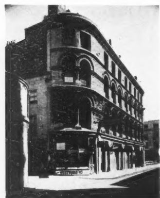
11, 1-2, St. Nicholas Street, Bristol, designed by Ponton and Gough and completed before 1867; note the free-standing iron columns in front of the shop windows.
