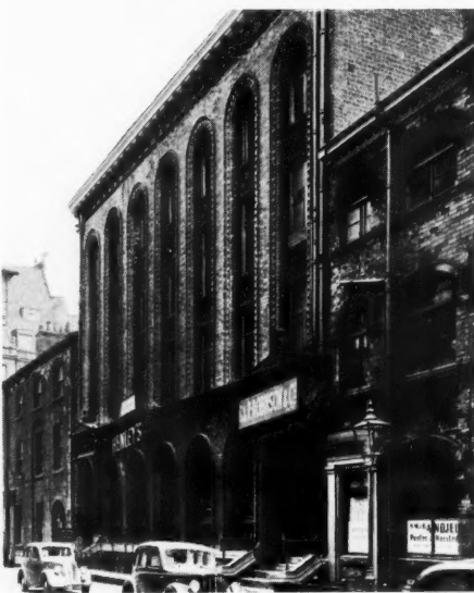
10, 59-60, Mark Row, London, designed by George Aitchison and built in 1864 for a real estate company for letting; in the facade of this iron-framed building the intradoses of the ground floor arches have heavy mouldings sinking into the plain piers and stilt blocks, to emphasize the thickness of the wall, while in the upper storeys the intradoses are plain, suggesting almost that the arcades stand free in front of the window plane. 11, 1-2, St. Nicholas Street, Bristol, designed by Ponton and Gough and completed before 1867; note the free-standing iron columns in front of the shop windows.
