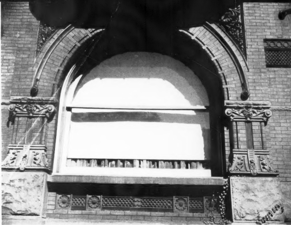
3, safety curtain: all the world's a stage. Convolutions of terra-cotta and brick give hint of mahogany splendours within.
