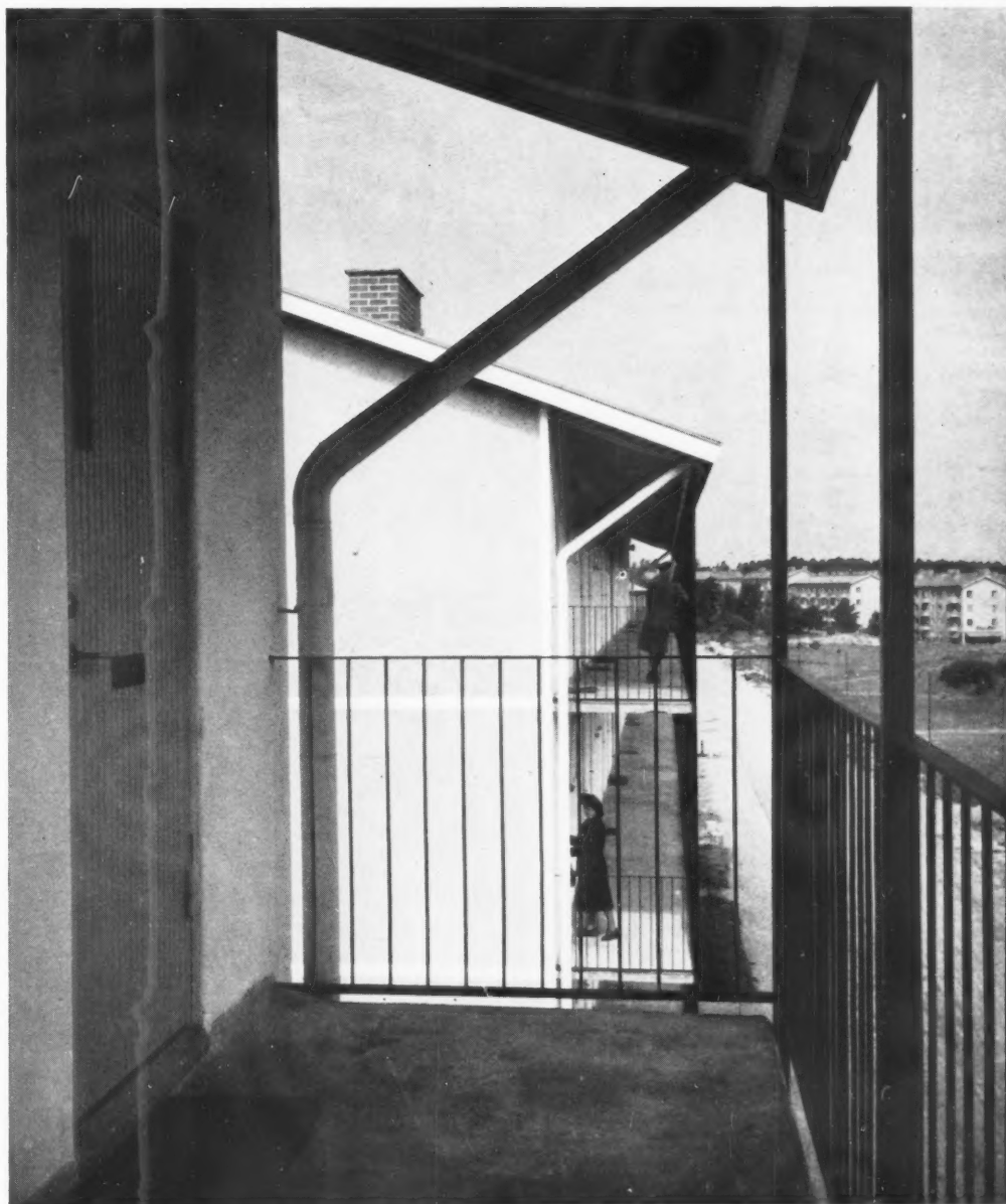
1. looking towards the south block from an apartment doorway.
