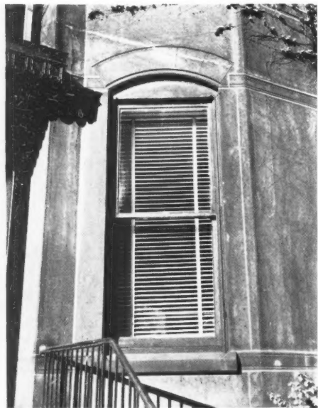
8, looking forward. Decoration limited to surface incisions, the wall, like the canopy, appears to be of pressed metal.
