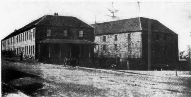
Commissariat Store, Sydney; construction began 1809. Building on right 1812, demolished 1939.
