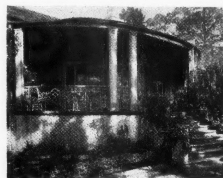
The curved verandah of Greystanes, Prospect Hill, N. S. W.
