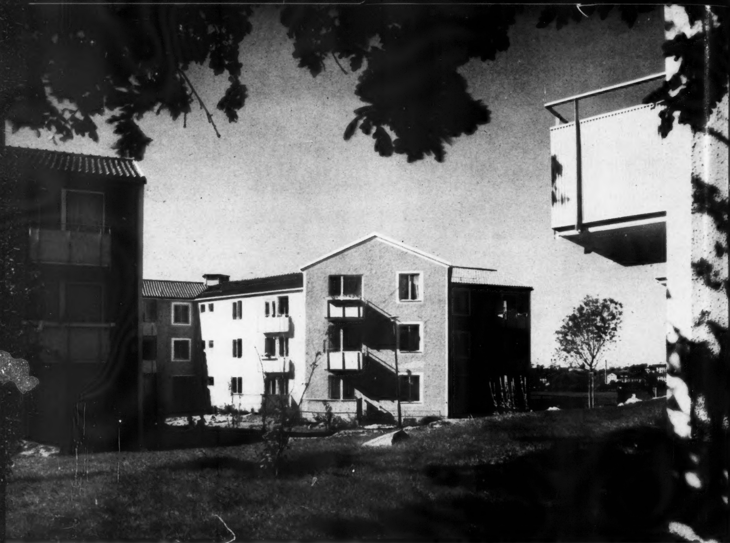
3, a view into one of the hexagonal courtyards formed by the conjoined star blocks. Lake Mälaren can be seen between the buildings.
