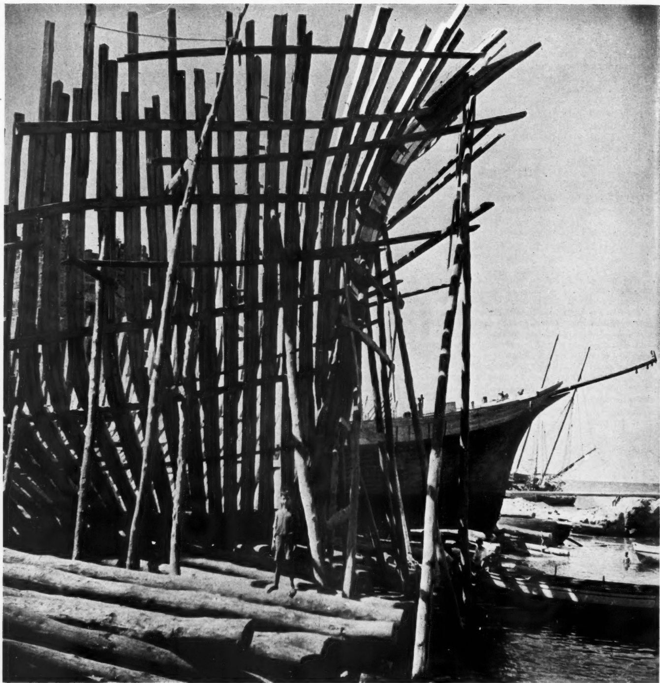
From every angle along Ruad's harbour-front and foreshore half-built skeletons of ships rear their timbers, or completed hulls lie ready for launching and fitting-out. Coasting schooners are the island's speciality. They are manned by the Ruadis themselves, who have a tradition of seamanship dating from the Phœnician period, and trade as far south as the ports of Egypt and north to Alexandretta and Asia Minor.
