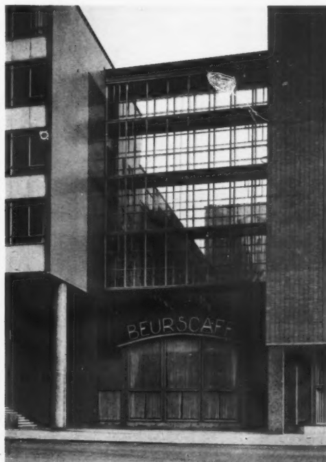
24, an entrance to the restaurant. The glass galleries above it join together the two main office wings.
