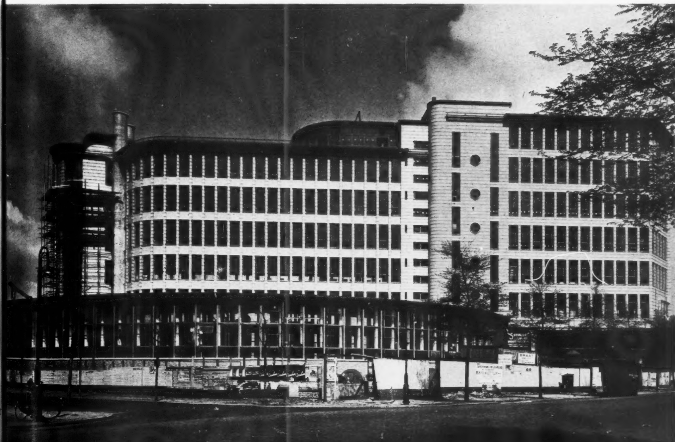
30, the insurance building from the south with the circular wing housing the company's files in the foreground, and the office wing behind.
