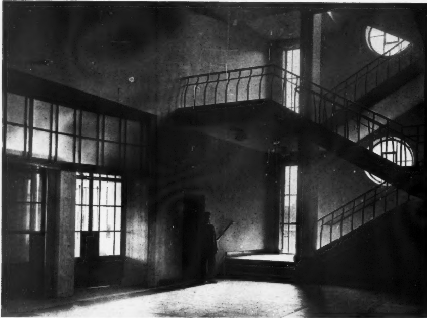
31, the main entrance hall of the insurance building, with the staircase serving the office wing.
