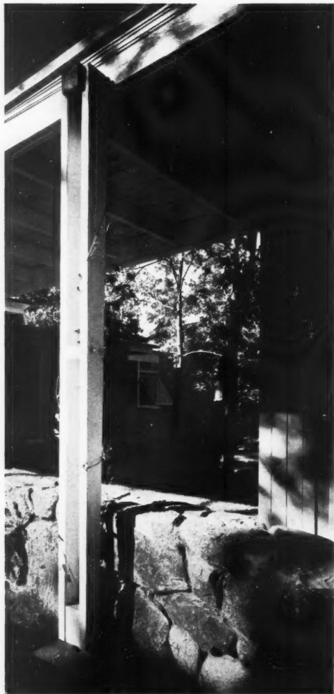
2. a detail of one of the posts supporting the covered way, which joins the garage to the rest of the house. The low wall is of local stone. 3, the covered way leading up to the front door, with a view through the house to the living terrace.
