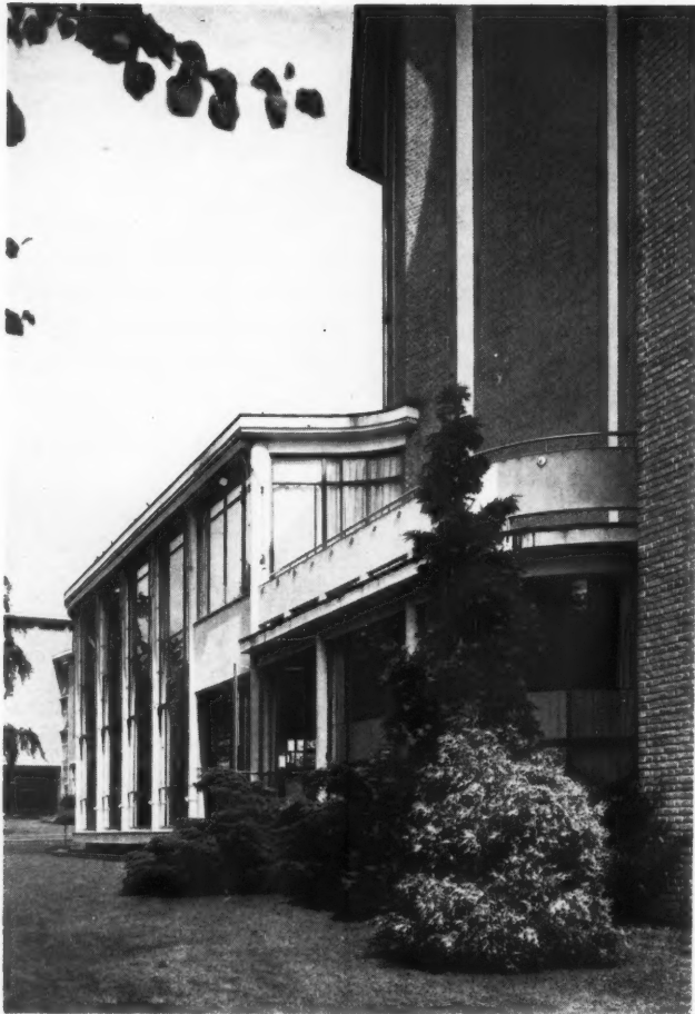
2, the exterior of the entrance hall and terrace to the new jazz band and orchestral studios, across a road from the earlier buildings.
