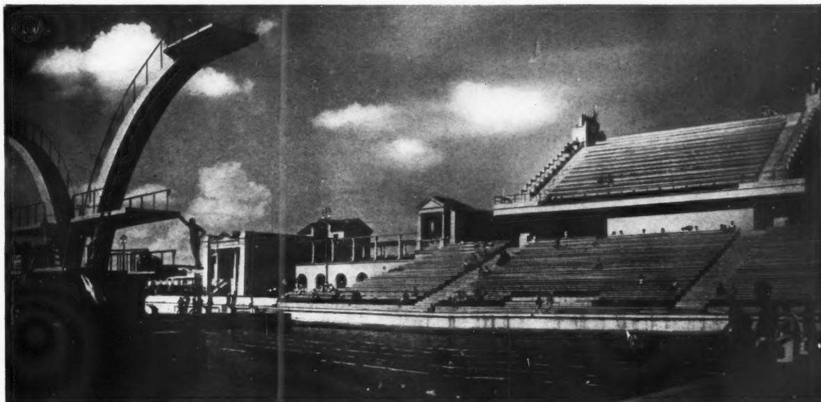
2, the Dynamo Aquatic Stadium at Khimki, Moscow, by Gennady Movcham, 1938. It is interesting to note that the contrast in architectural expression of the classical pavilions, classical pergolas and classical symmetry altogether with the bold construction of the grand-stand and the diving boards, apparently did not worry the architect.
