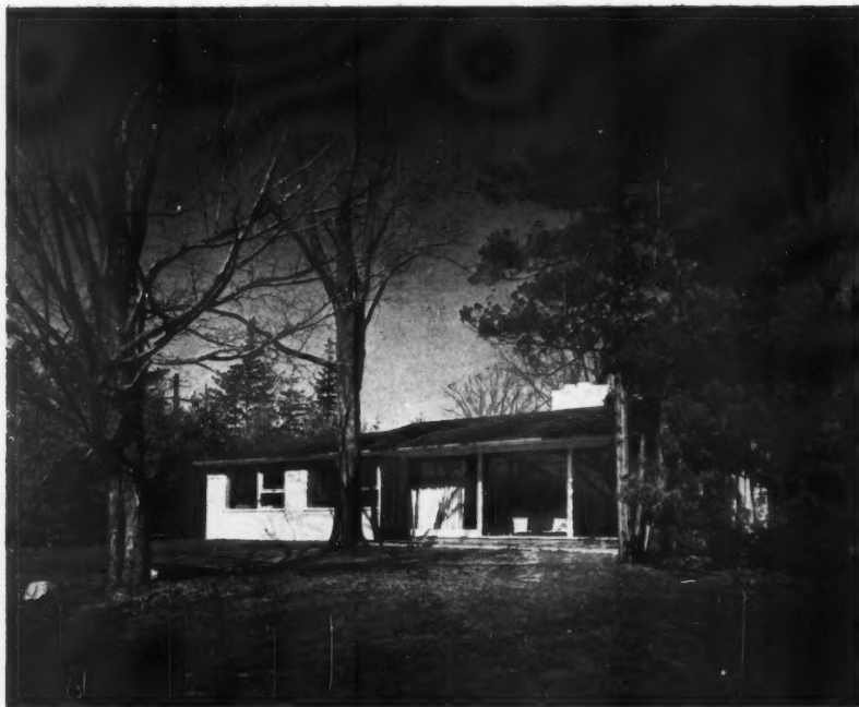
4, the house from the south-east, showing its relation to the trees on the site. 5, the living room, with the sliding dining table half out.
