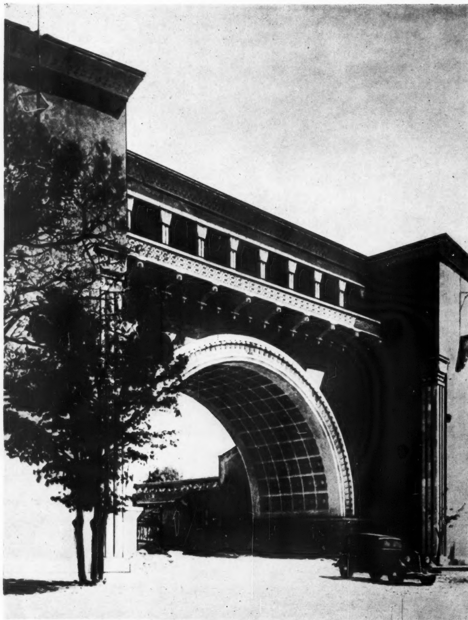
3, the Dynamo Stadium, Tbilisi, by Archil Kurdiani, 1939. As bewildering a contrast as in the previous pictures—but this time not between Classical and Functional but between a regional Monumental and the classical Monumental of Roman coffered vaults. The piers in the corners are the places where the two sets of motifs meet. An attempt at understanding this and similar contrasts would probably have to take into account the fact that the reactions to architecture of the man-in-the-street are of necessity more associational than visual. If his wishes are the architect's laws, as they are in Russia, then he has no reason not to continue what is reminiscent of imperial grandeur and of local lore. Objections on the grounds of aesthetic incompatibility are considered formalism (as against realism).
