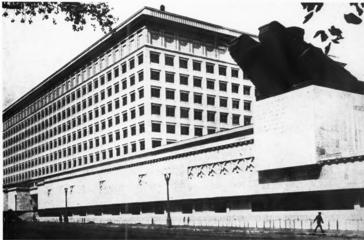
1, the Frunze Military Academy, Moscow, by Lev Rudnev and Vladimir Munz, 1937. A remarkable combination of elements—the main block of a type first developed in America about 1890, and then by men such as Behrens in Germany: a utilitarian structure crowned by a few very restrained classical elements. The ground floor screen on the other hand is bare, forbidding and wholly of a twentieth century monumental style, including its inset ornamental panels which succeed in making of hammer and sickle a pattern reminiscent of Paris and Western Avenue. The tank is a monument to the purpose of the building as well as to socialist realism in sculpture.
