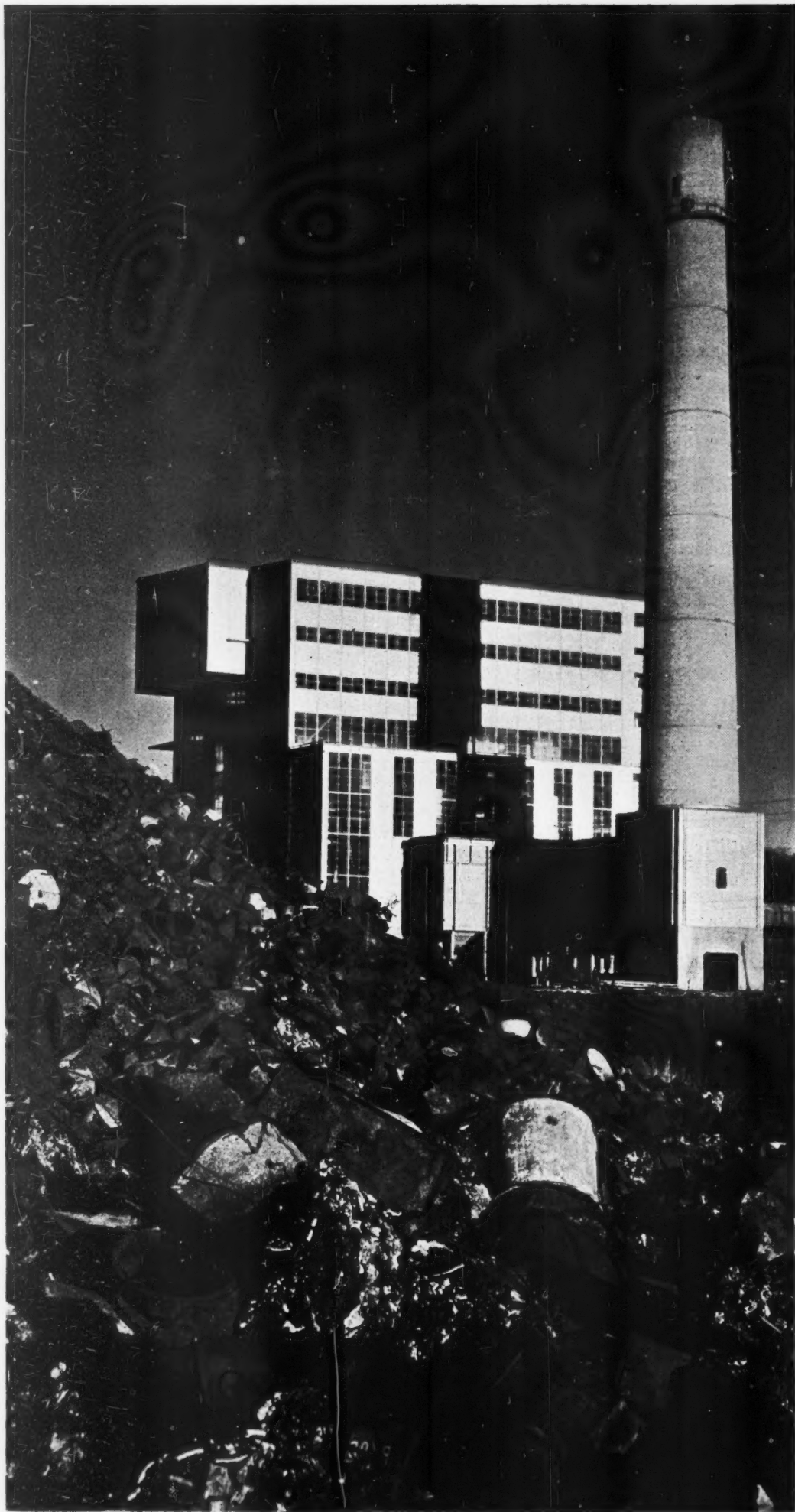
STOCKHOLM INCINERATOR PLANT
