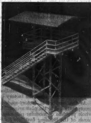
Model of a framed wood structure by a second year (first term) student.
