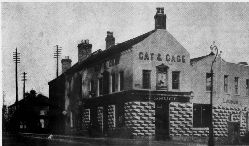
The main front and the undulating side-wall of this pub are decorated with mock-rustication in which, for no very obvious reason, the depth of the stones increases course by course, from the plinth up. A detail is shown on page 26.
