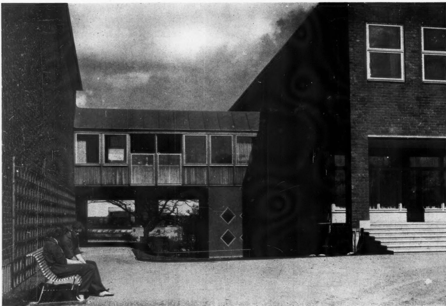
2, a detail of the communicating corridor between the administration building and the gymnasium. All the windows slide vertically and the panels are of impregnated redwood. This corridor achieves a lightness and originality of design that goes some way towards countering the tendency to staidness elsewhere.
