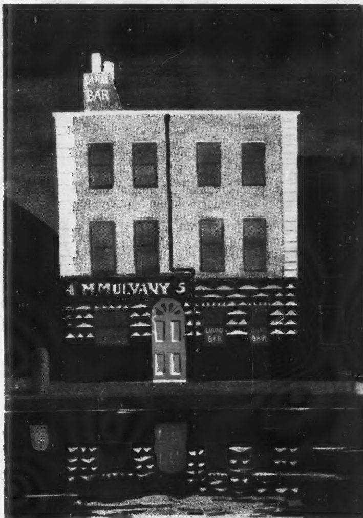
The Canal Bar in Dublin faces the canal running to the Guinness works. It is surrounded on all sides by nineteenth-century warehouses and factory buildings, which although satisfactory enough in design are undeniably sombre in tone. The lozenge-work is of particular interest as the usual relationship of dark to light has been reversed, producing an illusion of reflected light, as from snow on the ground.
