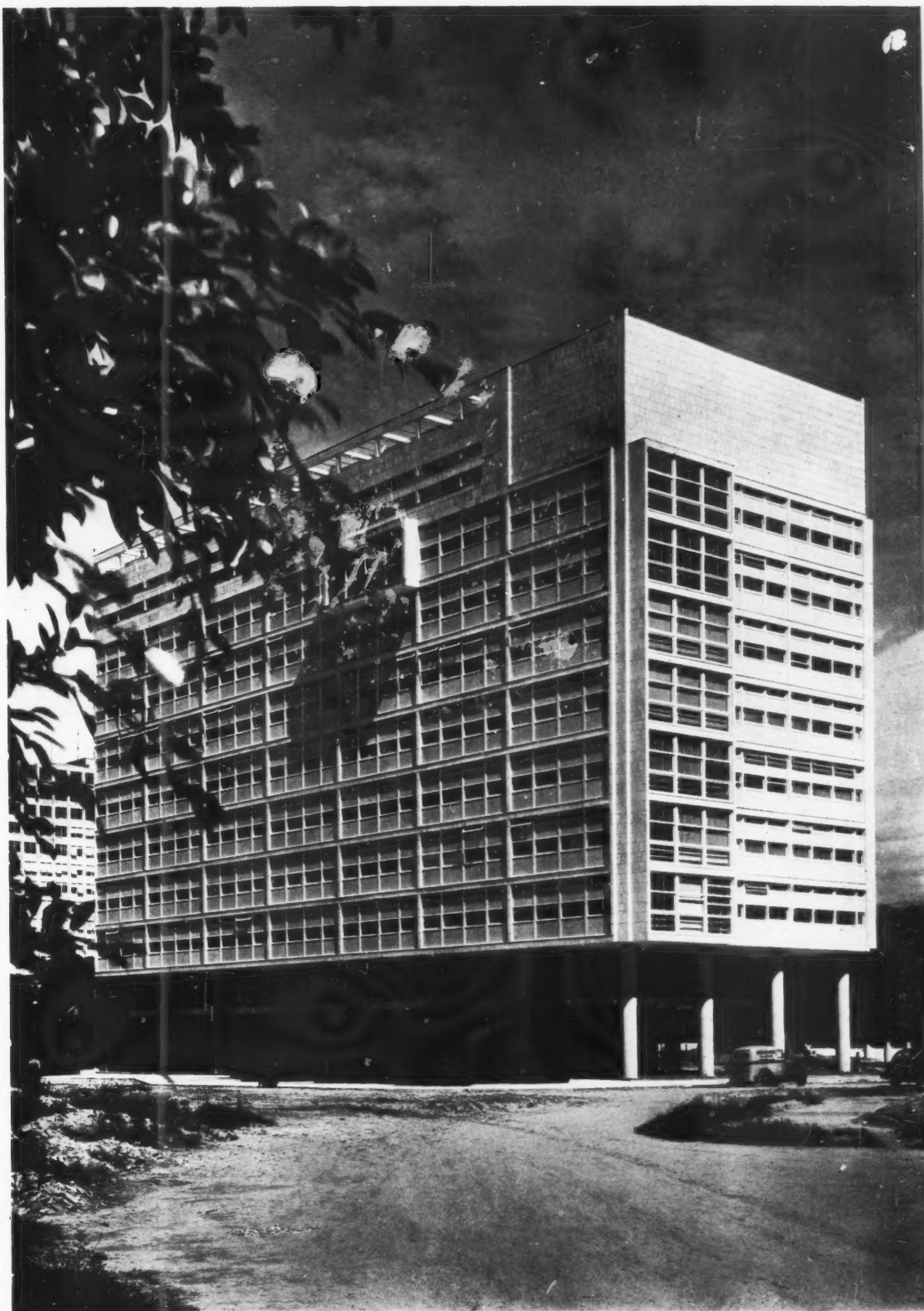
1. the I.R.B. building from the south-east. The standardized wall-window panels are wood-framed.
