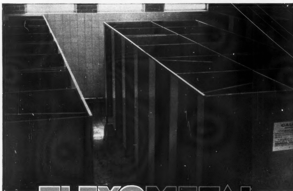
Above: Solid laminated Flexometal doors completely sealed in steel, at the Chorley Baths, Lancashire. Below: Photograph showing the saving in space effected by the use of Flexometal for dressing cubicles. Architect: Percy Howard, A.R.I.B.A.
