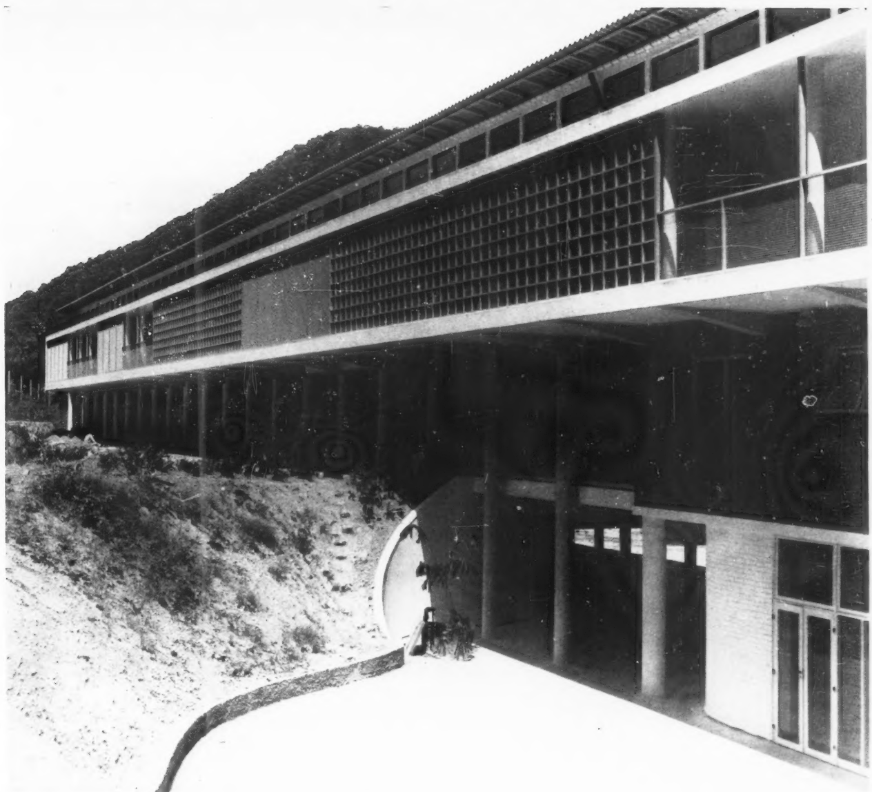
1, the south façade, facing the hill, with the main entrance to the building.
